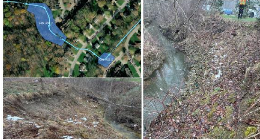
Aurora Shores Erosion & Flooding
