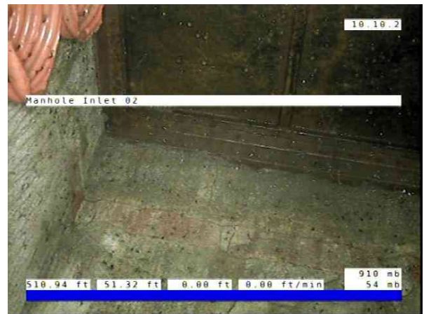
Inlet02-Inlet 03_aa85427d-9380-416e-bf6a-99993cae7bd0_20251010_085 809_833.jpg, 00:04:43, 51.32ft Manhole / Inlet 02
