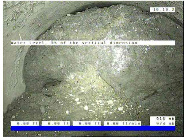
Inlet04-Inlet 05_0b6b54d4-1ae0-4886-a919-0bd9db447a9c_20251010_100 721_453.jpg, 00:00:03, 0.00ft Water Level, 5% of the vertical dimension
