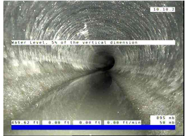
Inlet02-Inlet 03_6cd41142-0efb-4015-8b6c-2e067fc3128f_20251010_0852 19_792.jpg, 00:00:03, 0.00ft Water Level, 5% of the vertical dimension
