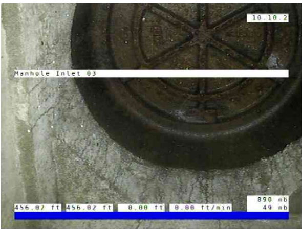
Inlet03-Inlet 04_d446c0f7-ca37-43ab-8d3c-f7ff7cd21453_20251010_08505 9_820.jpg, 00:21:13, 456.02ft Manhole / Inlet 03
