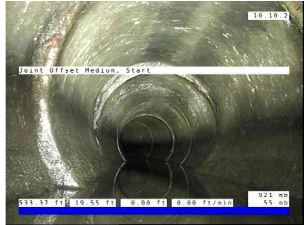
Inlet01-Inlet 02_b087f79d-6333-44a5-aa5c-0431f36e8aa6_20251010_0903 02_990.jpg, 00:02:20, 19.55ft Joint Offset Medium, Start
