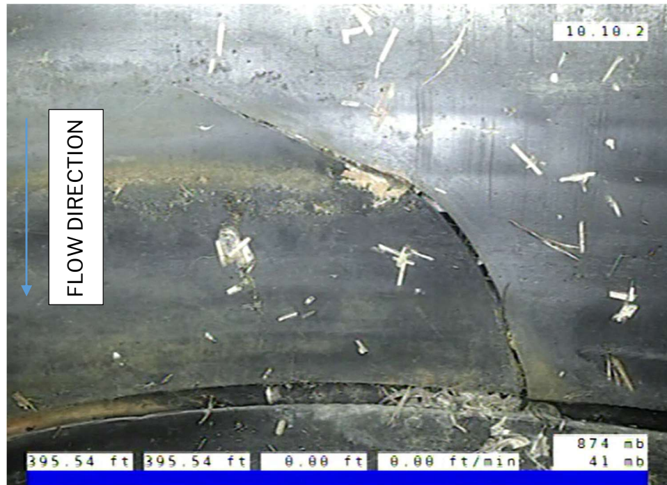
Figure 3: Perforation of corrugated metal pipe section
