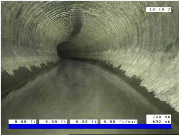
Inlet03-Inlet 04_98847996-b37f-4dea-af19-56fe634cb99e_20251010_0822 15_261.jpg, 00:00:00, 0.00ft Catch Basin / Inlet 04
