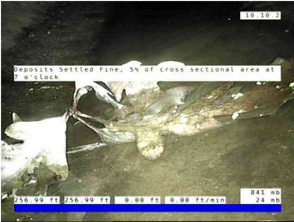
Inlet03-Inlet 04_9a3dac02-c805-4a2b-acf4-5ed19167fc32_20251010_0838 25_603.jpg, 00:10:26, 257.00ft Deposits Settled Fine, 5% of cross sectional area at 7 o'clock
