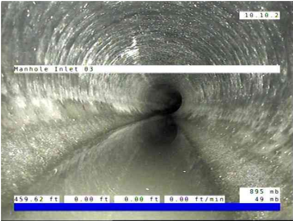
Inlet02-Inlet 03_bf241c86-e28c-4c86-b9c5-b242dc8ddb64_20251010_085 213_290.jpg, 00:00:00, 0.00ft Manhole / Inlet 03
