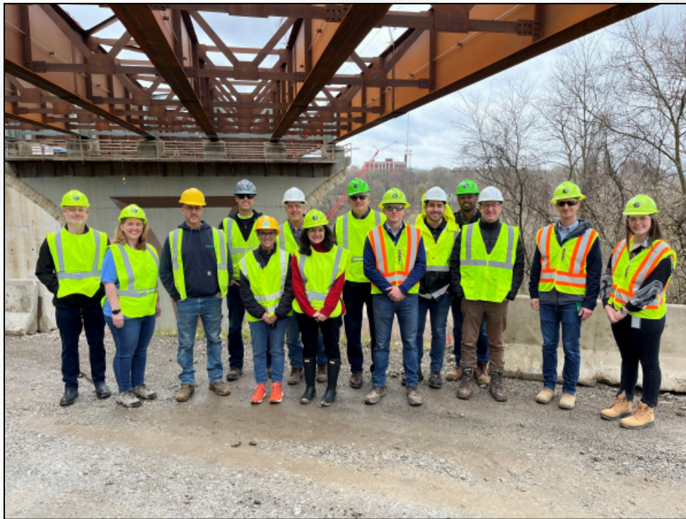
Representatives meet under the newly set Rt 8 Bridge superstructure
