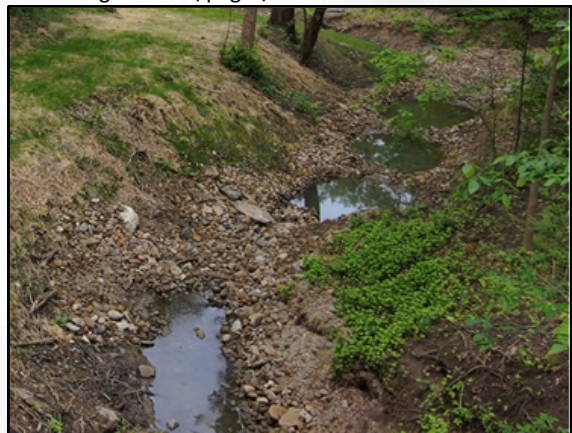
Wye Rd In-Stream Step Pools
