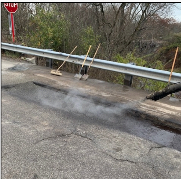
Hudson Run Road over Wolf Creek - BAR-007-0142
