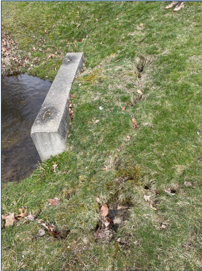
Figure 15. Erosion and slumping behind headwall.
