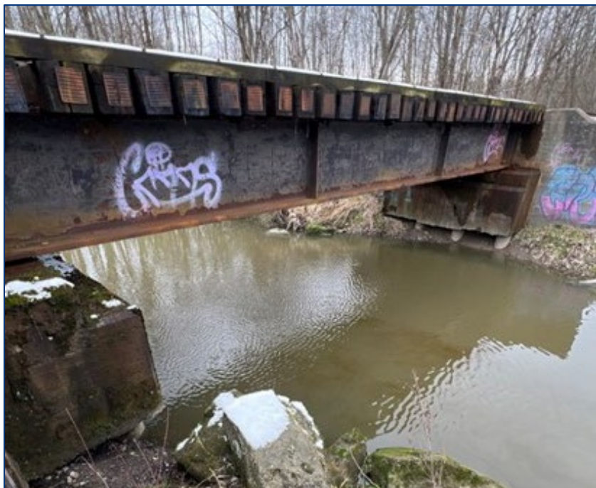
Figure 30. Railroad bridge with undercut abutment.
