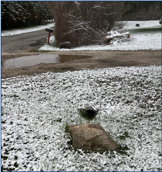
Figure 9. Partially blocked driveway culvert.
