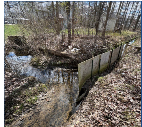
Figure 21. Homemade revetment with culvert outlet of tributary in background.
