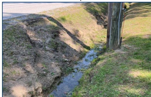
Figure 14. Erosion of roadside ditch
