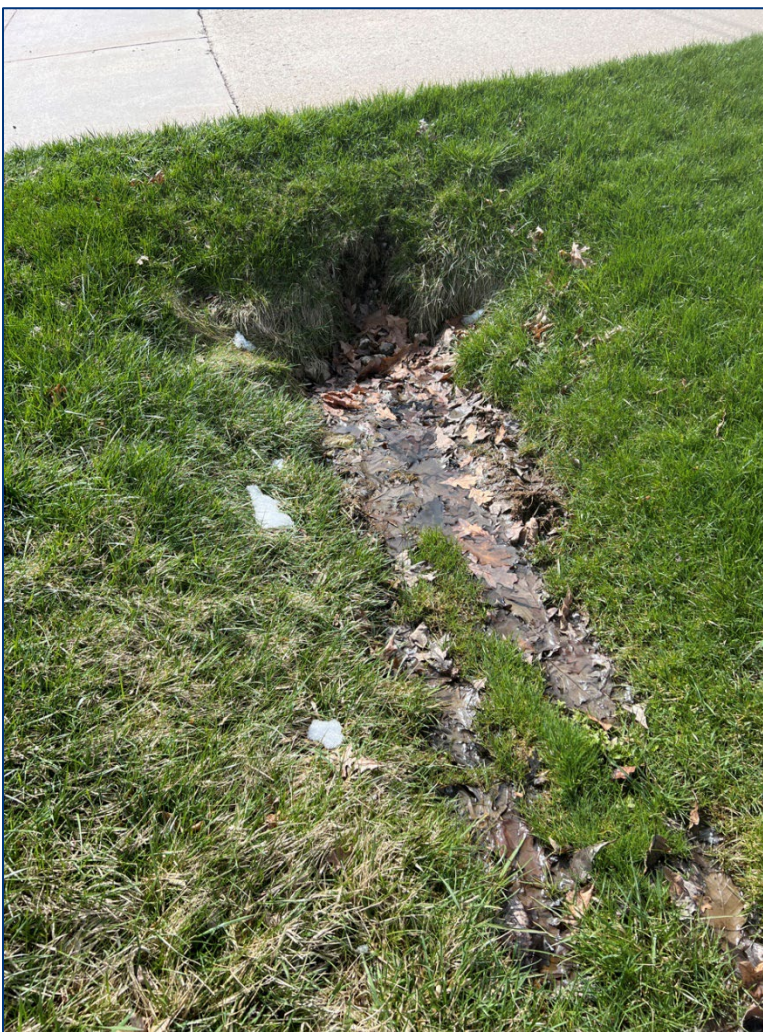
Figure 16. Blocked driveway culvert.
