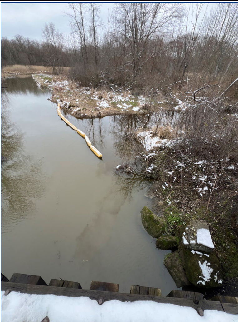
Figure 33. Containment boom on Pond Brook.
