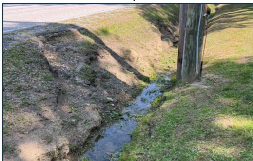
Figure 14. Erosion of roadside ditch
