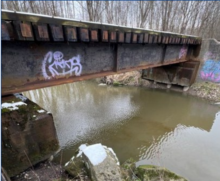
Figure 30. Railroad bridge with undercut abutment.
