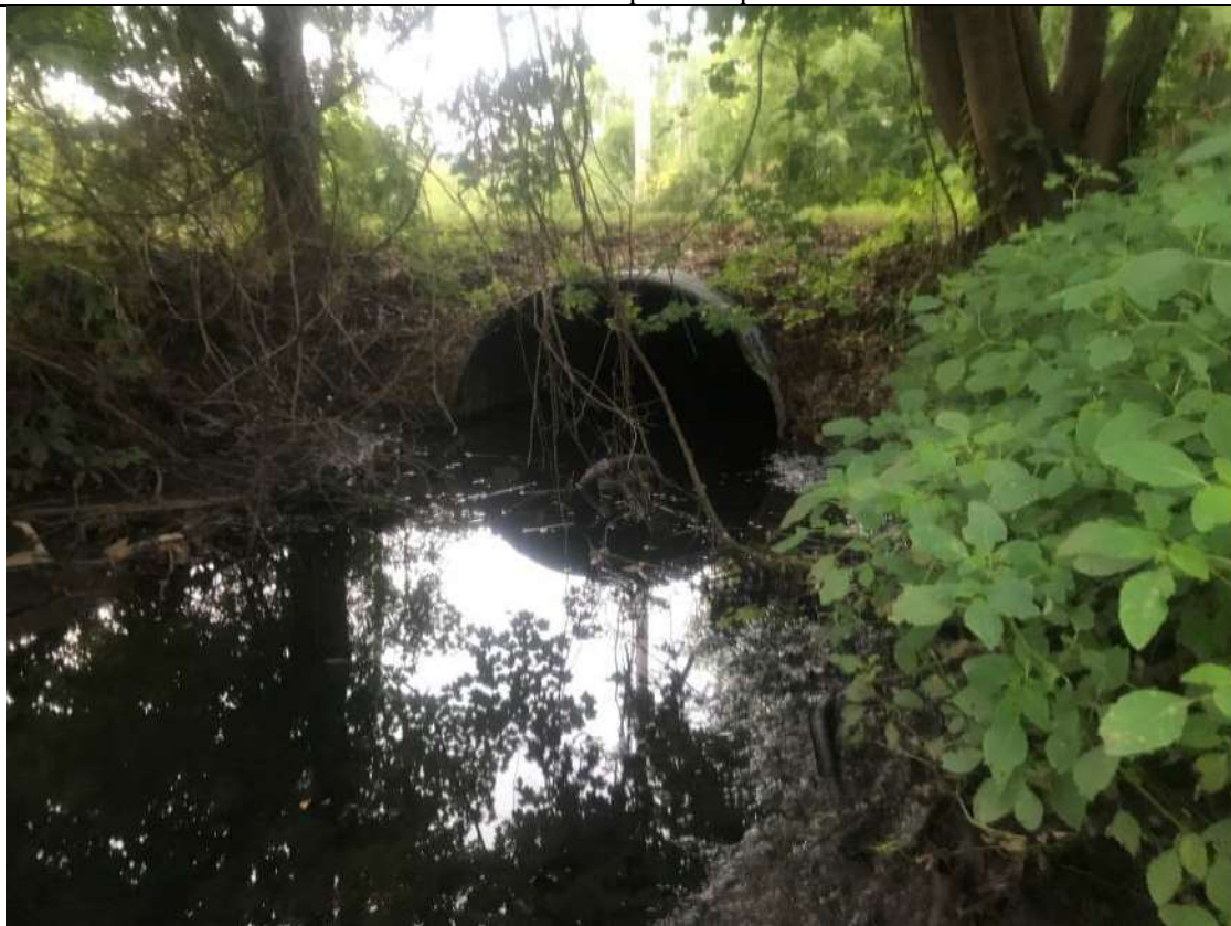
Photograph No. 12 STA 108+80 Downstream photo of 8ft CMP
