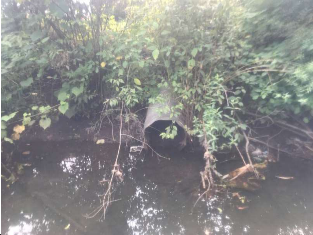
Photograph No. 9 STA 108+30 18" CMP on East side of creek
