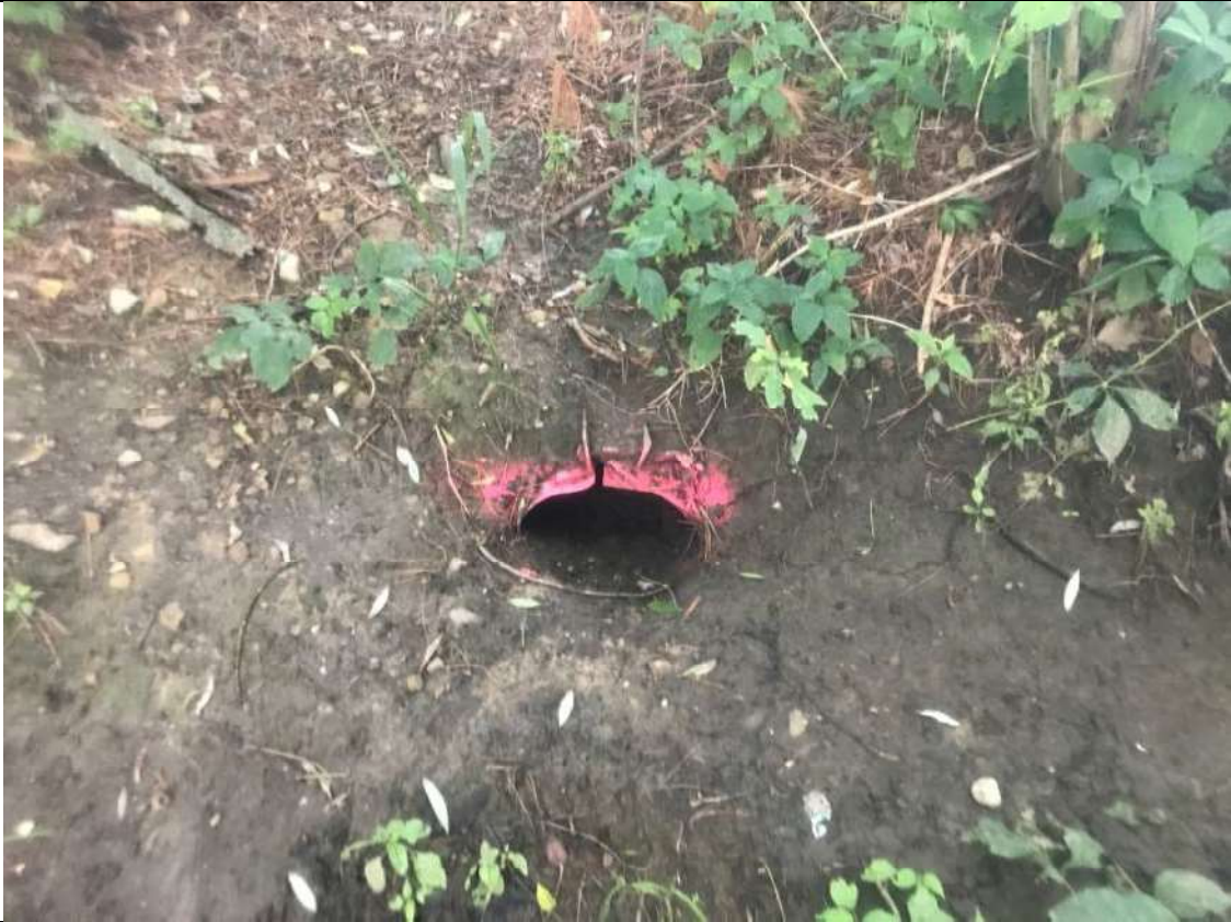
Photograph No. 37 Conceptual Plans STA 26+50 12" CMP
