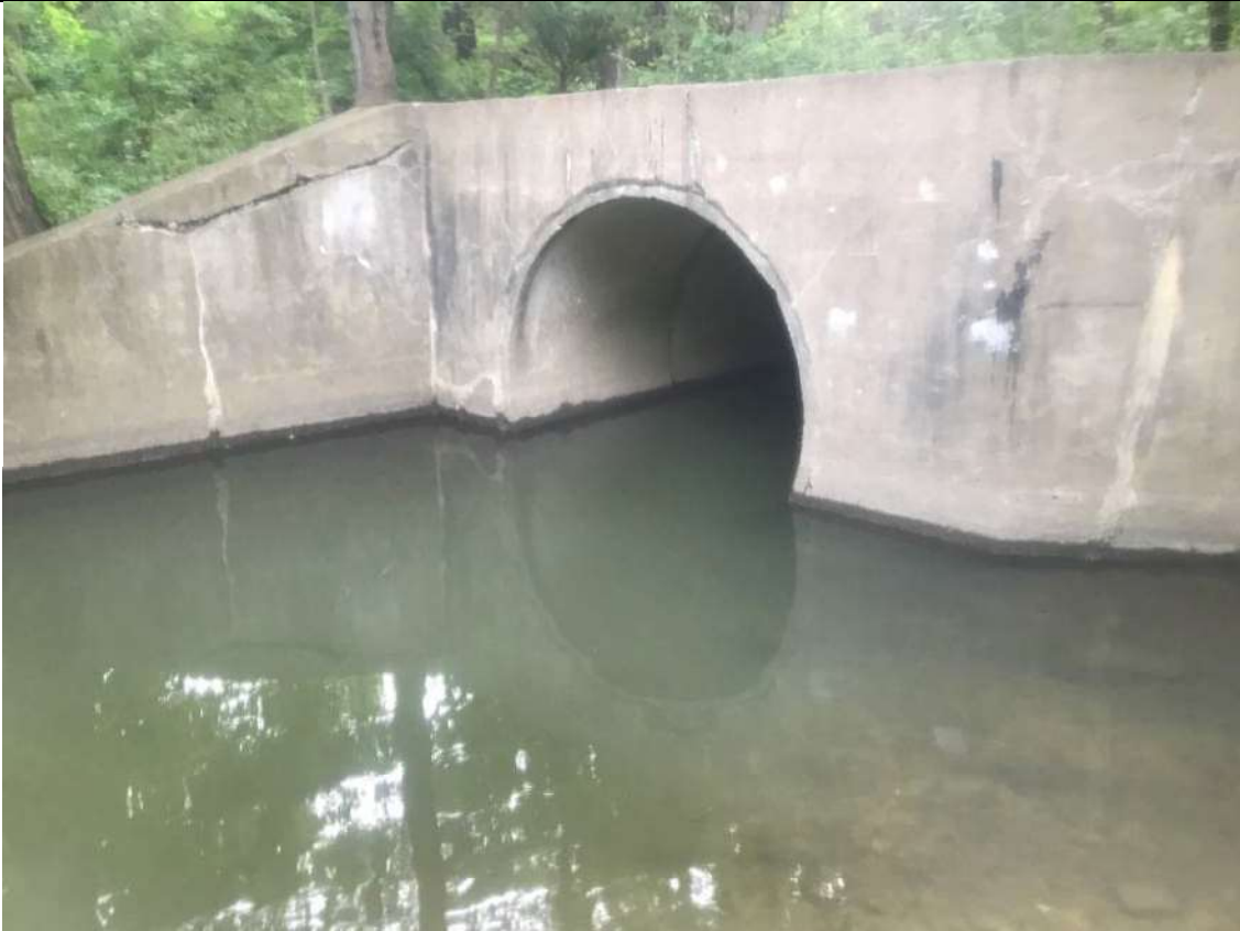
Photograph No. 65 Conceptual Plans STA 48+50 72" RCP on East side of creek
