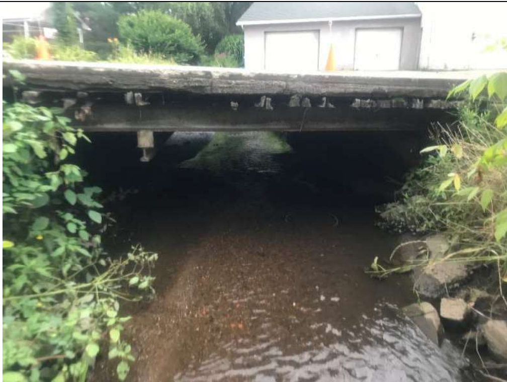
Photograph No. 17 STA 111+80 Downstream photo of bridge (18ft wide by 34" tall)
