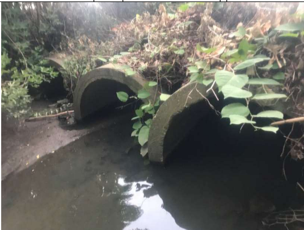
Photograph No. 14 STA 110+80 Downstream photo: 3 RPCs
