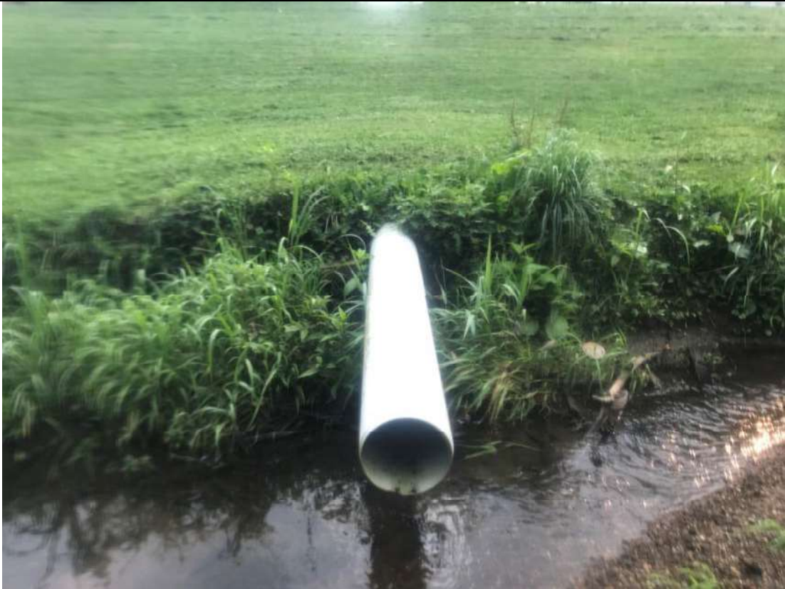
Photograph No. 50 Conceptual Plans STA 34+00 8" PVC on East side of creek
