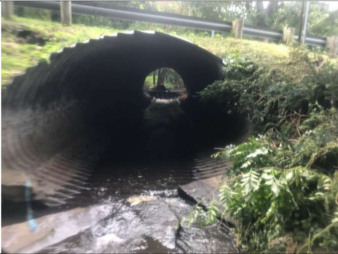
Photograph No. 69 Conceptual Plans STA 51+50 Upstream photo (11.5ft wide by 7'4" tall road crossing)
