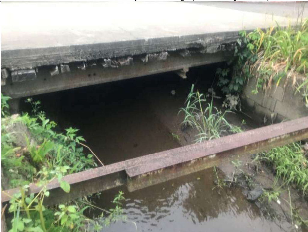
Photograph No. 18 STA 111+80 Upstream photo of bridge (18ft wide by 34" tall)
