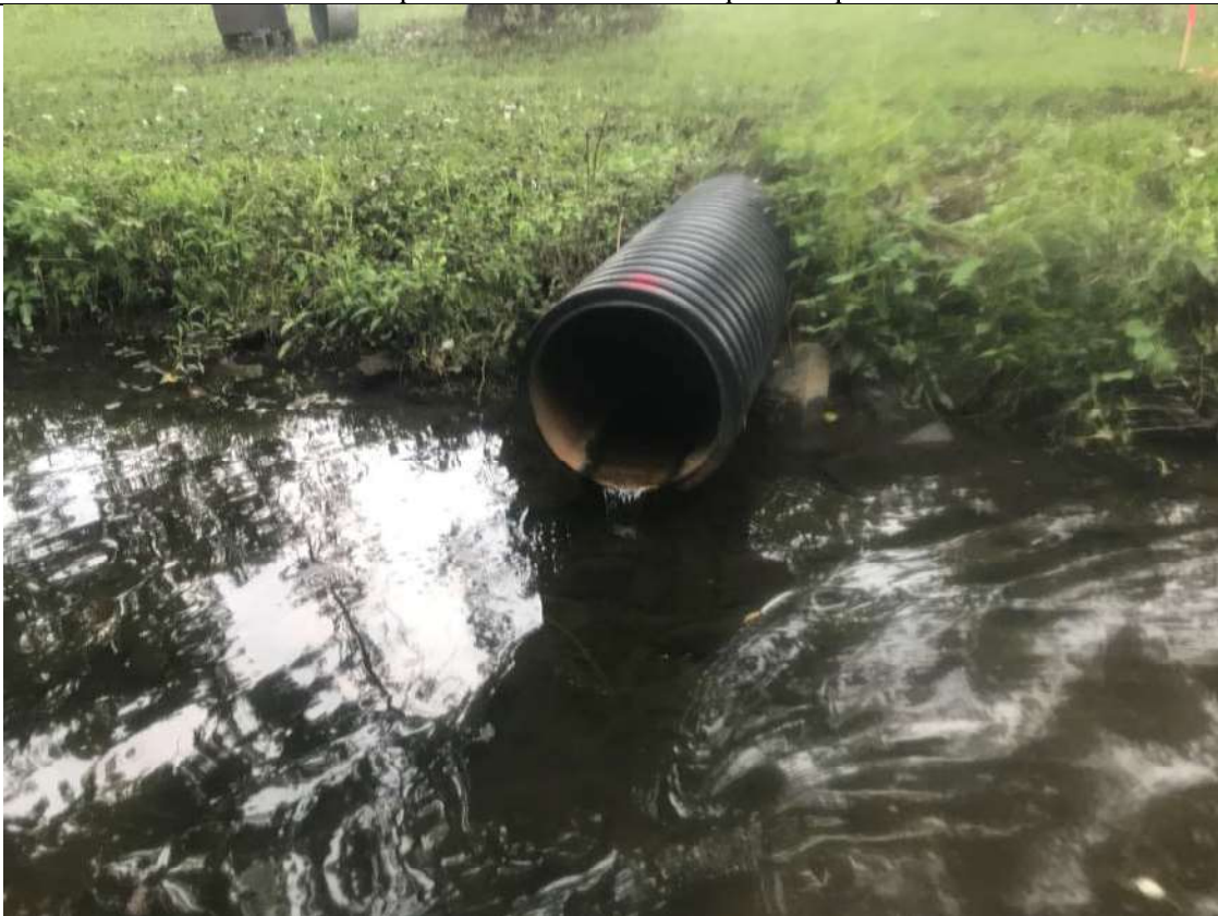
Photograph No. 44 Conceptual Plans STA 30+75 18" CPP
