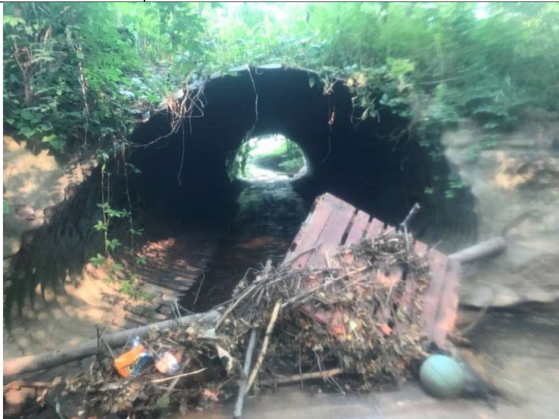
Photograph No. 66 Conceptual Plans STA 51+00 Downstream photo (11.5ft wide by 7'4" tall road crossing)
