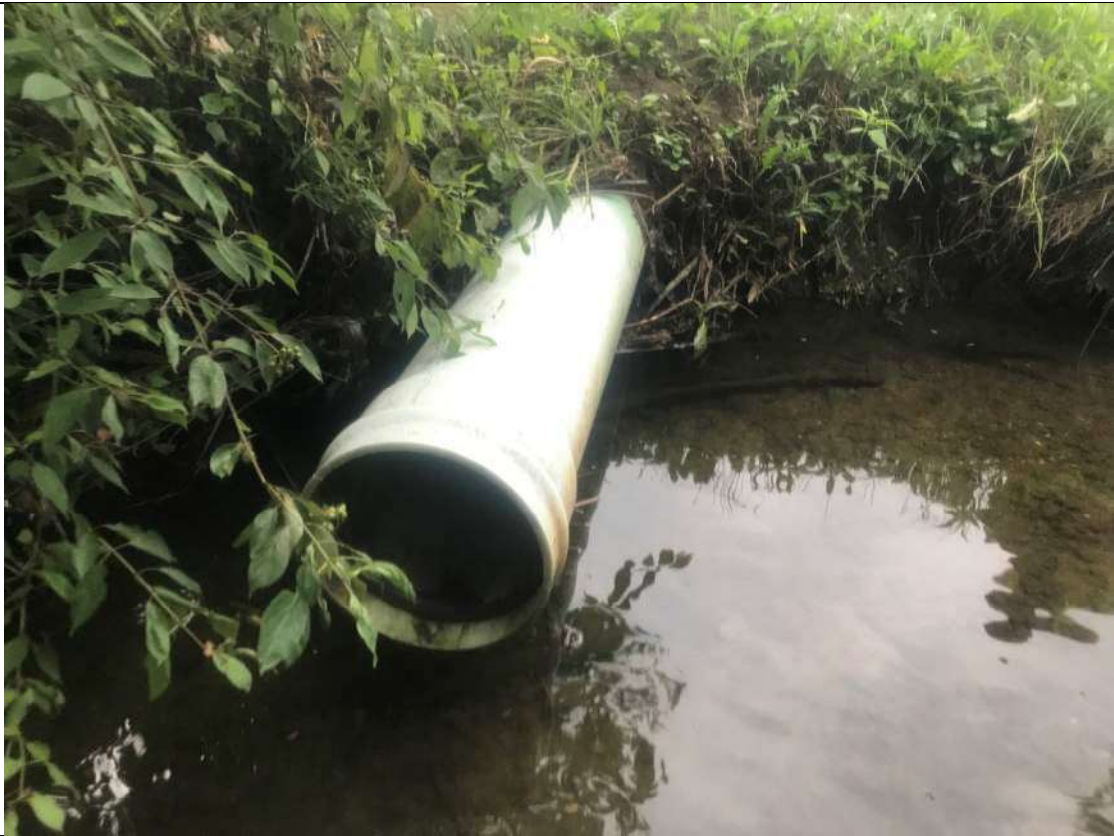
Photograph No. 41 Conceptual Plans STA 29+50 12" PVC
