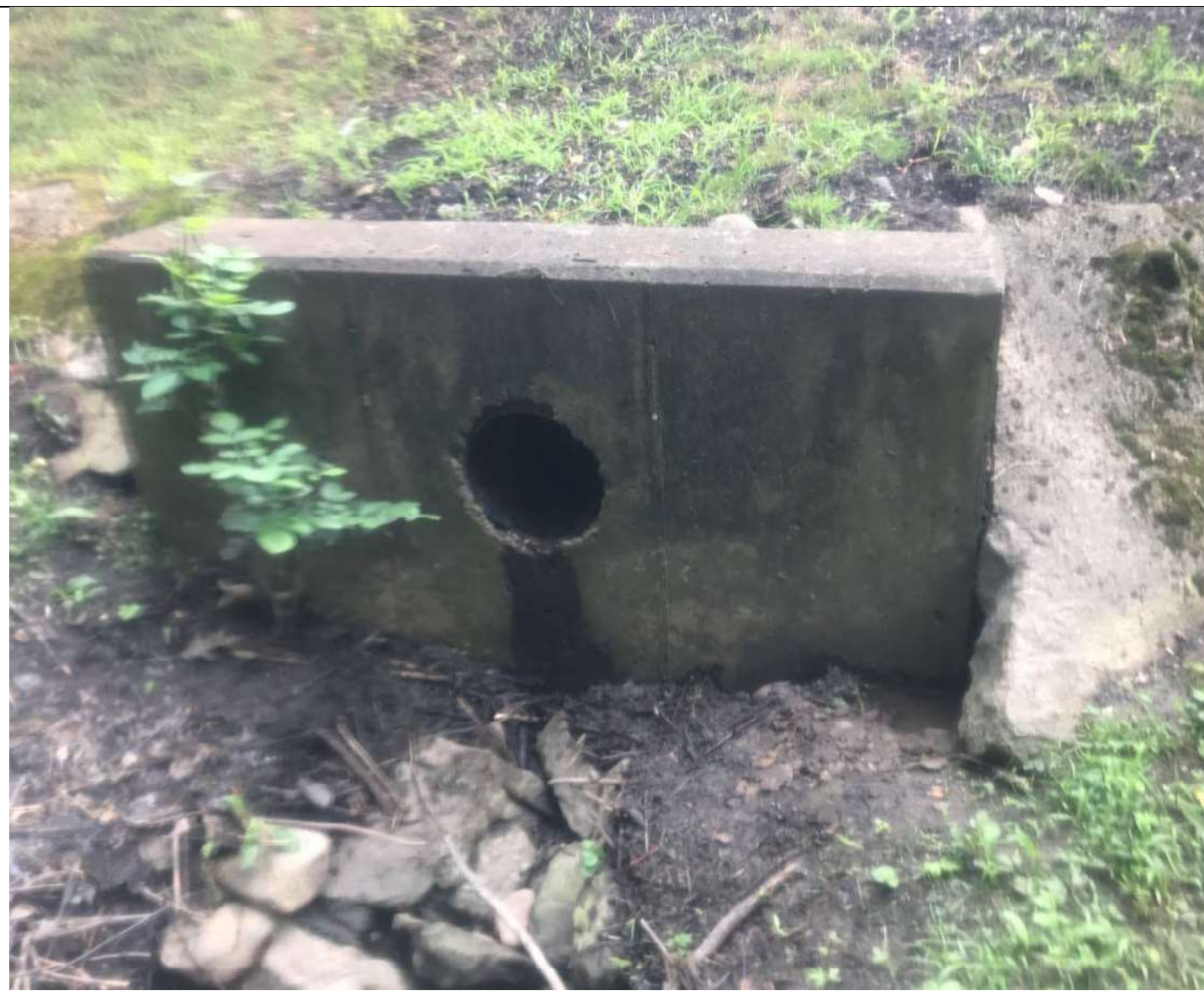
Photograph No. 75 Conceptual Plans STA 56+00 12" metal pipe just past county line
