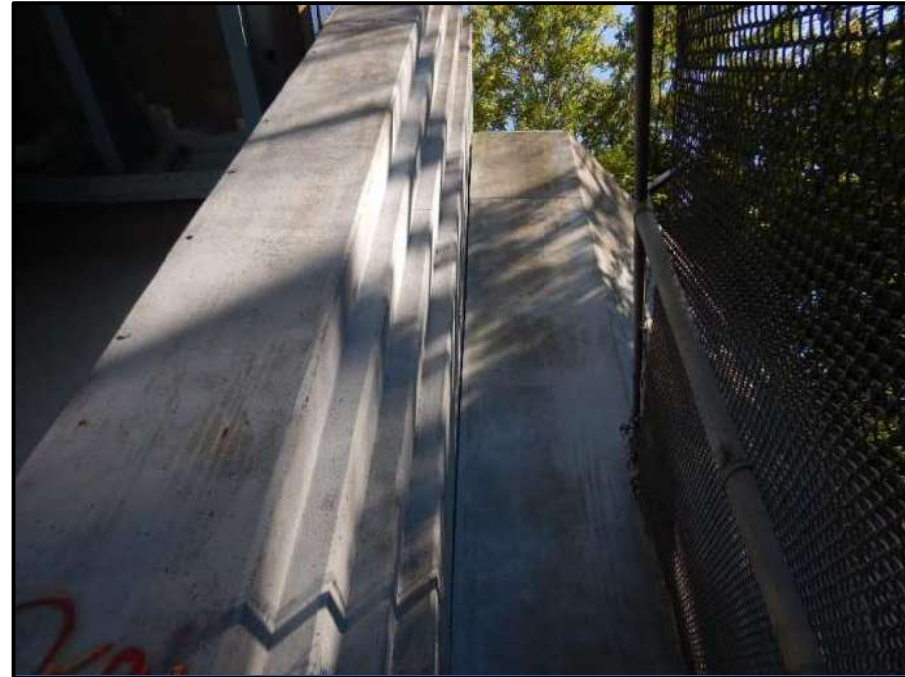
Photo 49 – Looking north at northeast wingwall at forward abutment. Note: wingwall rotation east away from abutment.
