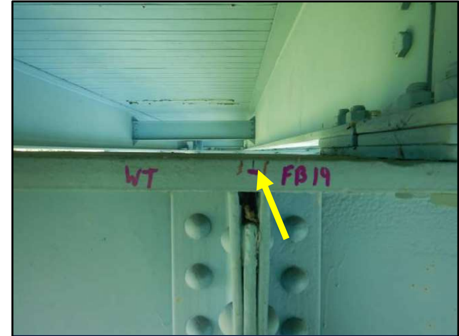
Photo 9 – Close-up of saw cut from 1991 rehabilitation project, south face of floorbeam 19 shown.
