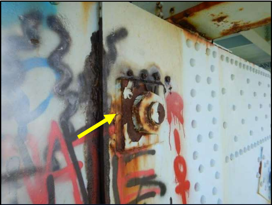
Photo 2 – Fillet welds along perimeter of hinge pin plate connected to U13 & U17 gusset plates.
