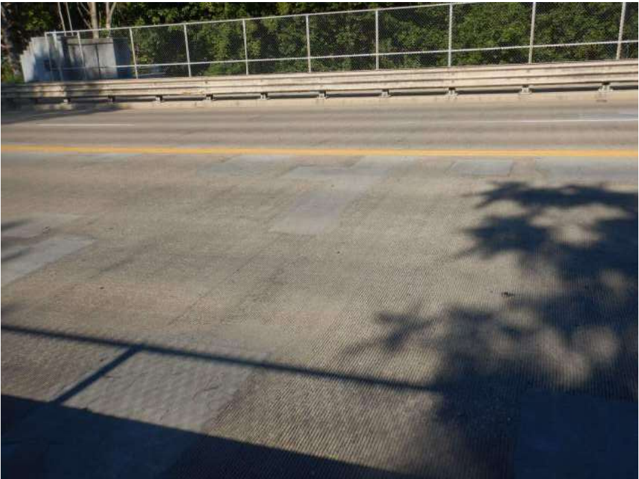
PHOTO 12 Condition Description Concrete patches in NB lanes, Span 1 shown, looking southwest. Note: Some patches exhibit cracking.
