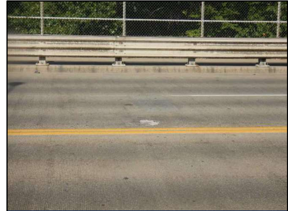
Photo 15 – Looking west at southbound lanes of bridge wearing surface near centerline, span 3. Note: 2 square-foot x 1-inch deep spall.
