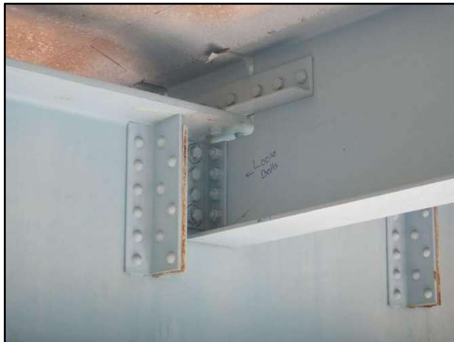
Photo 26 – Looking northeast at stringer 8 connection angle to south face of floorbeam 28, span 3. Note: two loose bolts.
