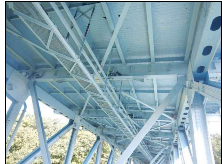
Photo 20 – Looking north at general underside grid deck in span 2. Note: isolated areas of surface corrosion in SIP forms.
