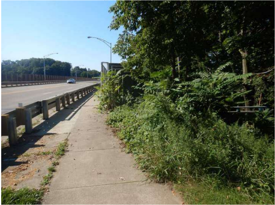
PHOTO 6 Condition Description Overgrown trees onto sidewalk at northwest corner, looking south.
