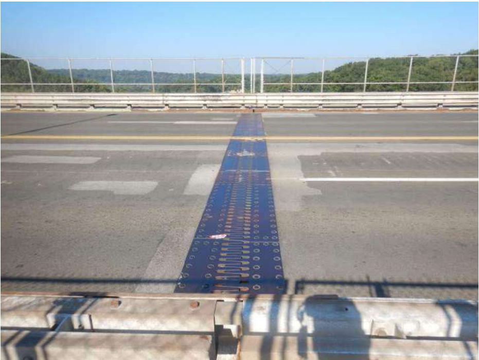
PHOTO 24 Condition Description Finger joint at Floorbeam 13, looking west.
