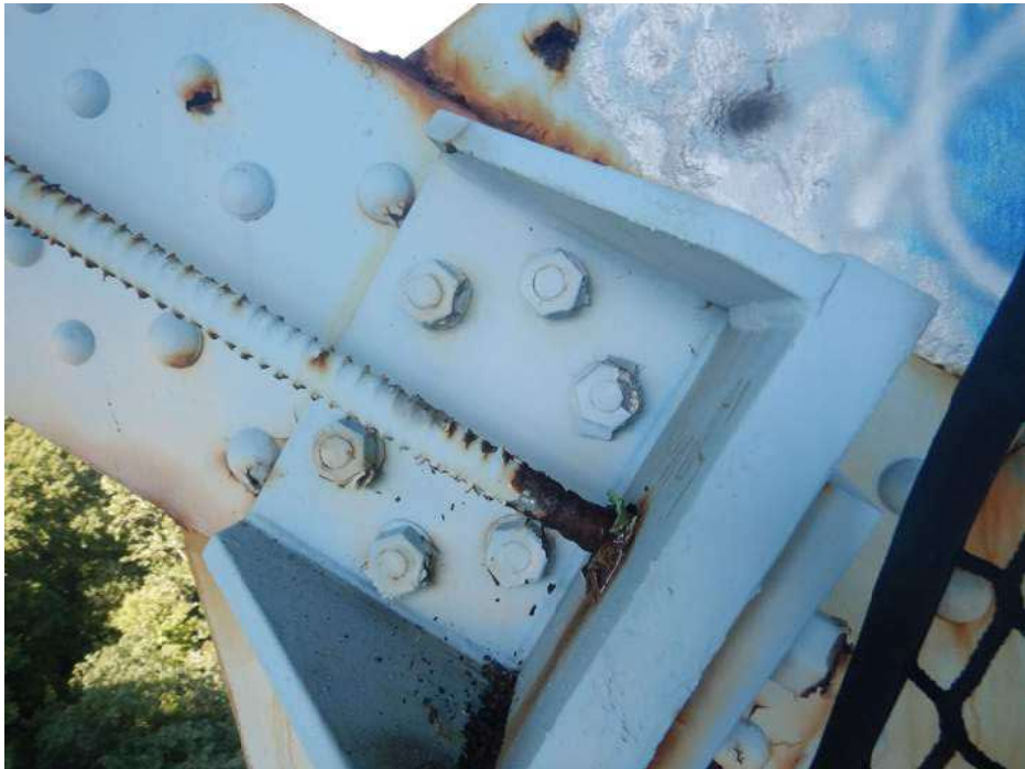
PHOTO 34 Condition Description PT rod exhibits moderate corrosion with up to 30% section loss, looking west at West U12L13.
