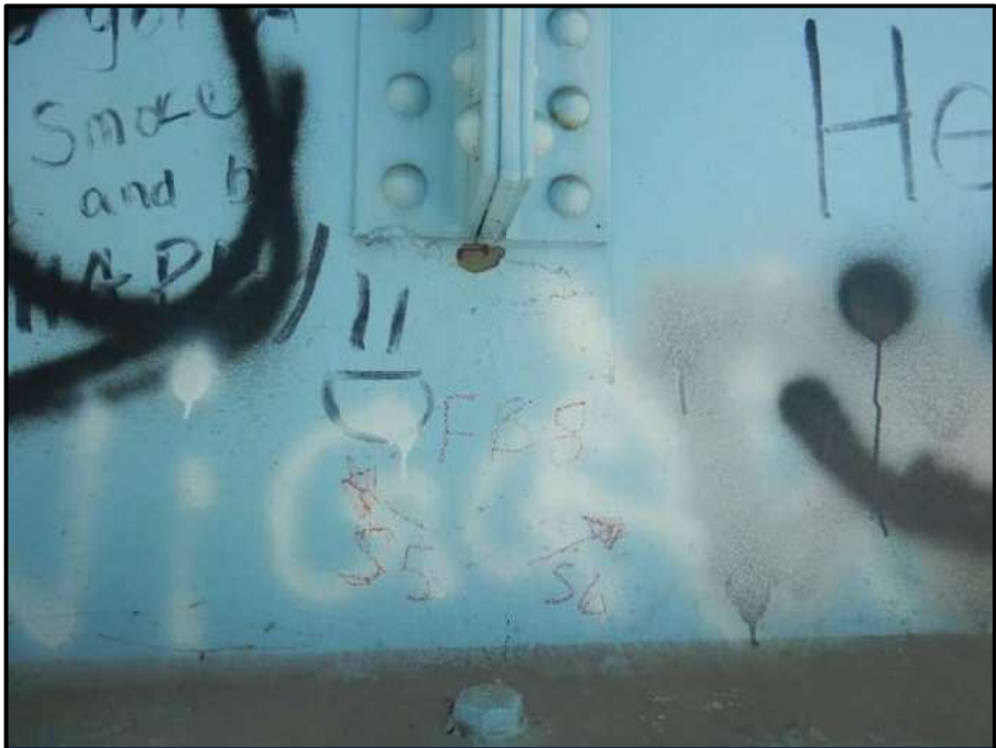
Photo 30 – Looking north at south face of floorbeam 8 under stringer 5, span 2. Note: minor cut in floorbeam web below stiffener. No change.
