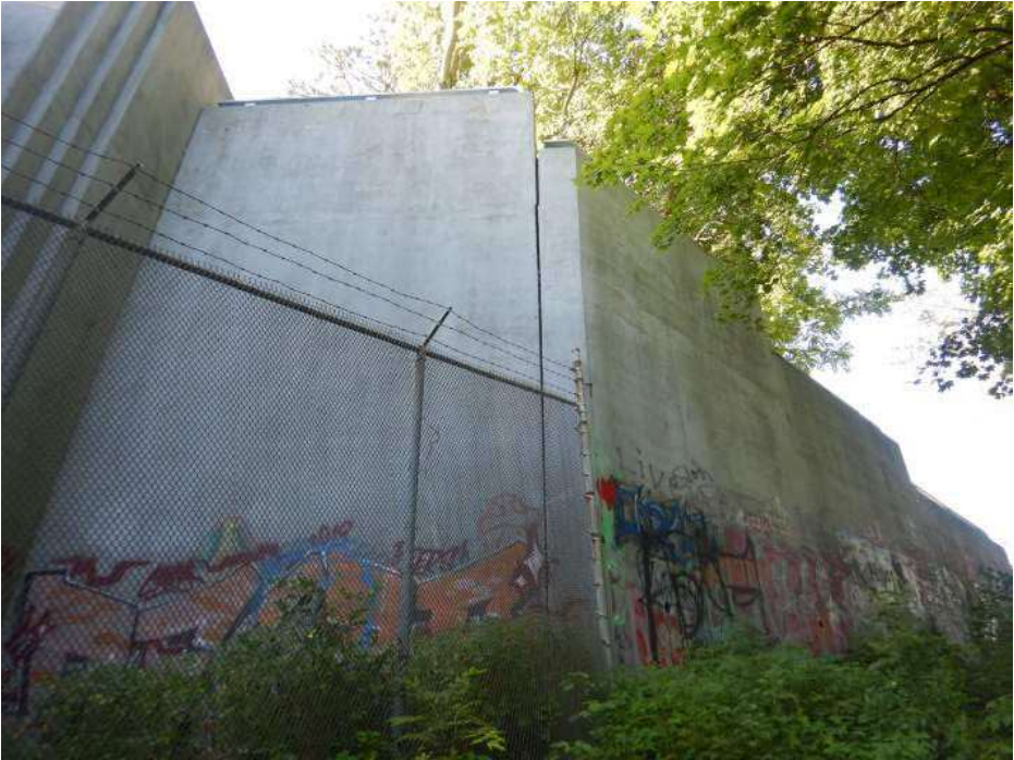
PHOTO 44 Condition Description Southwest wingwall rotating away from Rear Abutment, looking south.
