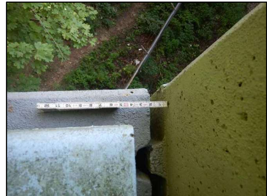
Photo 48 – Looking north at top of southwest wingwall Note: 1 3/4 inches rotation away from abutment.
