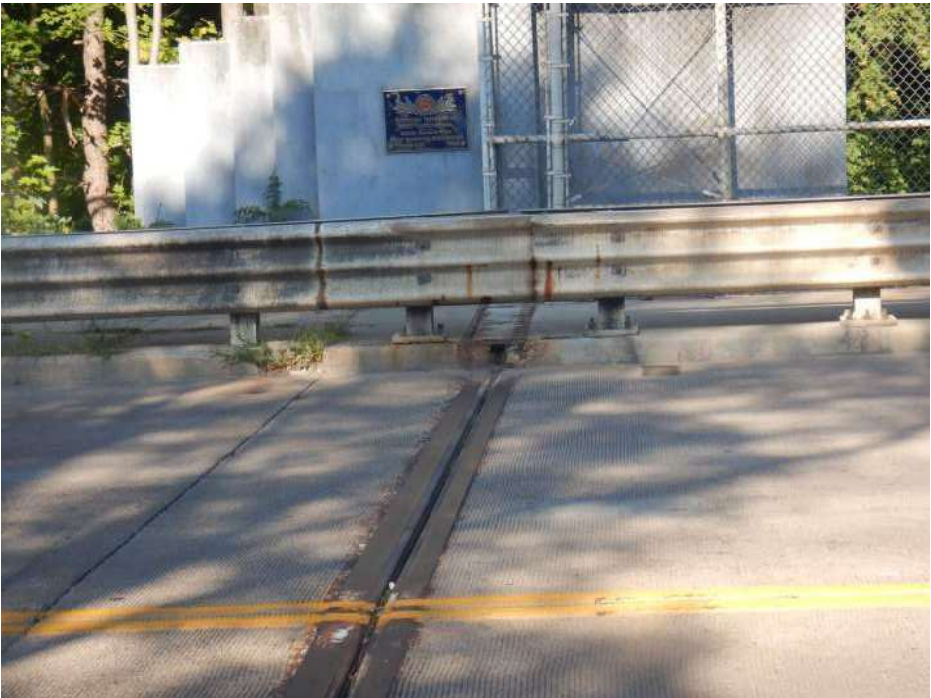
PHOTO 20 Condition Description Spalling in curb at at end of Rear Abutment joint, looking west.
