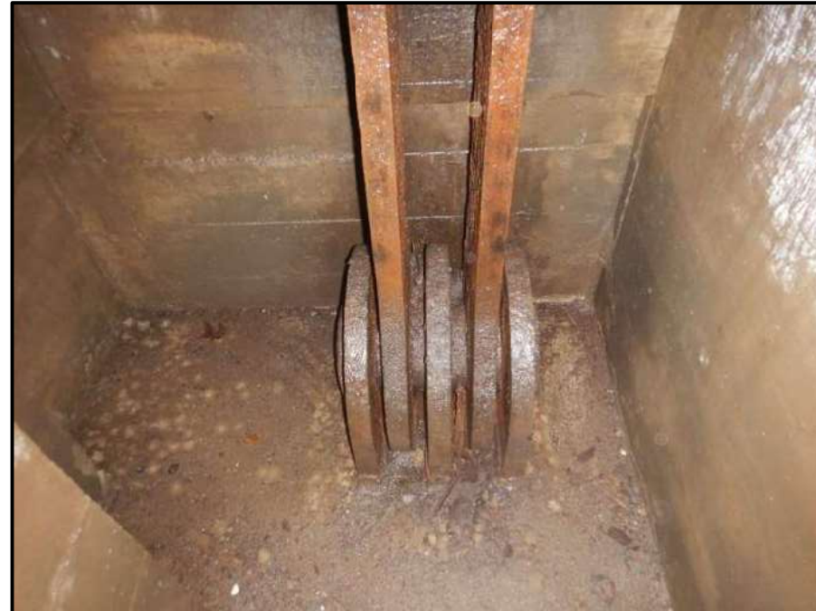
Photo 41 – Looking north at west truss anchor pit for tie down anchorage at forward abutment. Note: moisture inside of pit.
