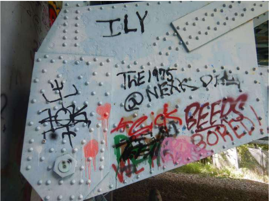
PHOTO 36 Condition Description Isolated areas of painted over pitting and section loss, looking west at OB gusset plate at East L0.
