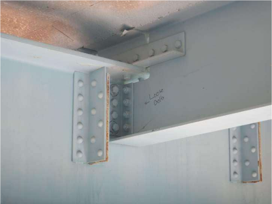
PHOTO 28 Condition Description Two loose bolts on Stringer 8 connection to Floorbeam 28, Span 3, looking northeast.
