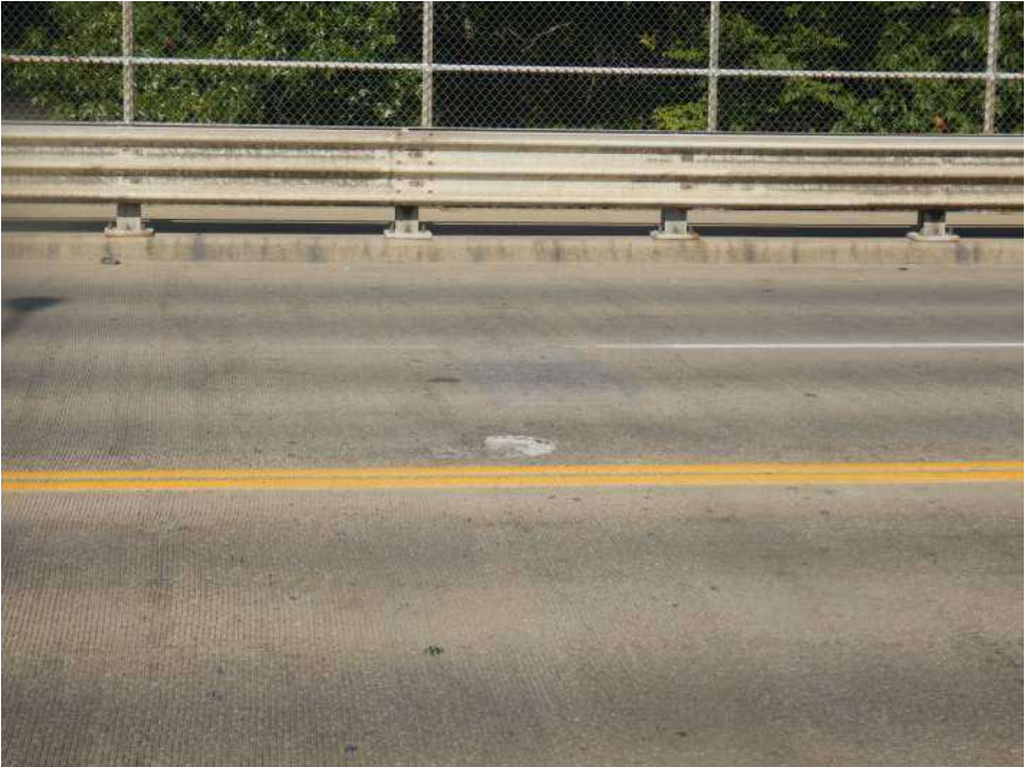
PHOTO 15 Condition Description 2-square-foot x 1-inch deep spall in SB lanes near centerline, Span 3, looking west.
