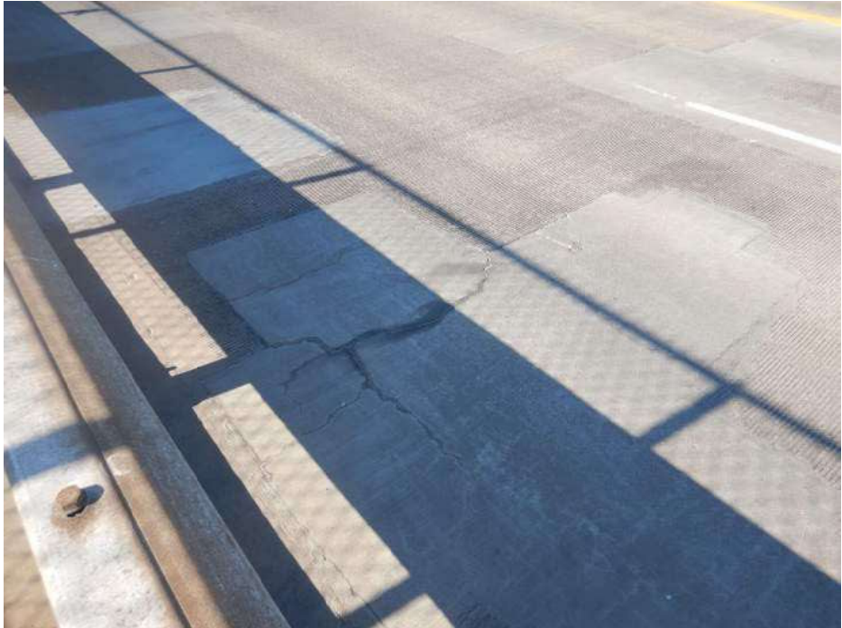
PHOTO 13 Condition Description Cracking in concrete patch in NB lanes of Span 1, looking southwest.
