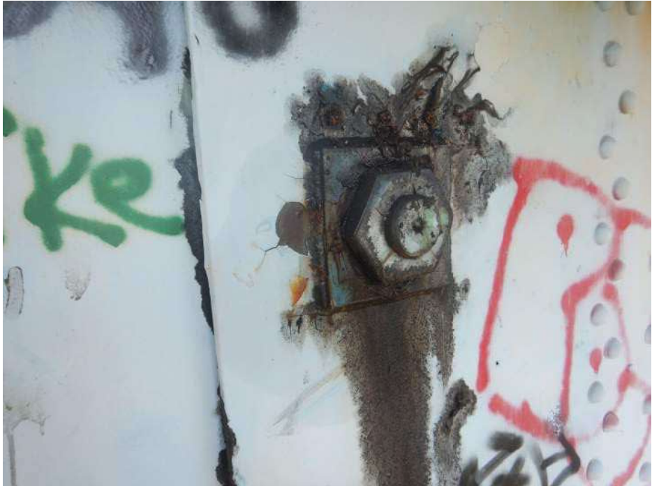
PHOTO 37 Condition Description Exterior pin and lomas nut connection on OB gusset plate, looking west at East U13. Note: No deficiencies in fillet weld. Pin heavily greased.
