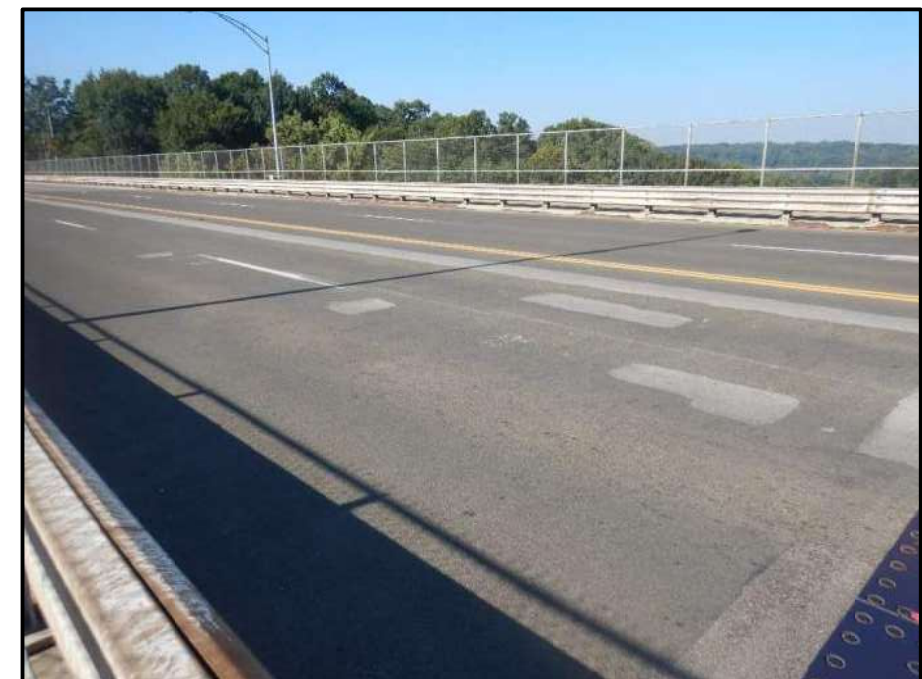
Photo 16 – Looking southwest at northbound lanes in span 2. Note: no change to epoxy overlay and patches in bridge wearing surface.
