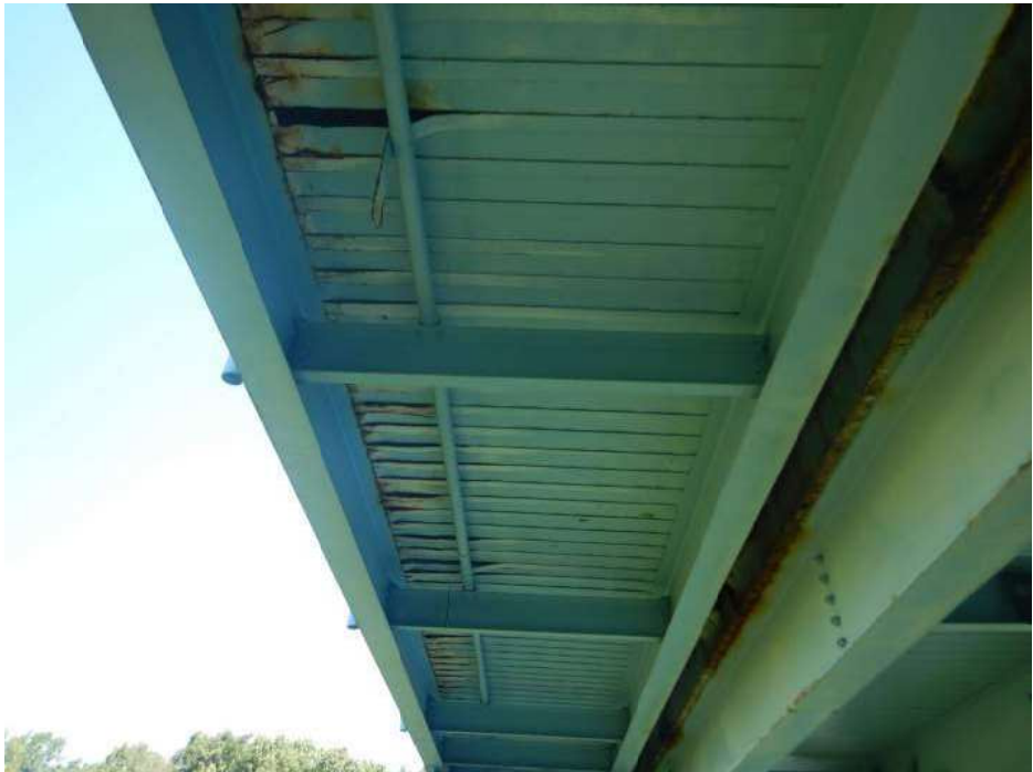
PHOTO 22 Condition Description Corroded SIP forms under west sidewalk in Span 2, looking north.
