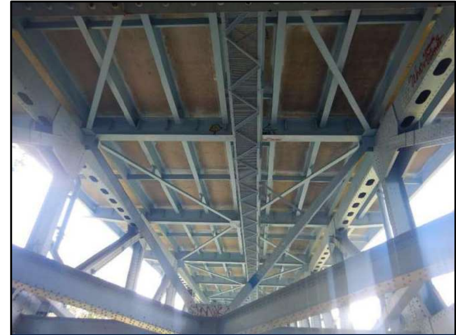
Photo 19 – Looking north at general underside of span 1. Note: cracking with light efflorescence in deck.
