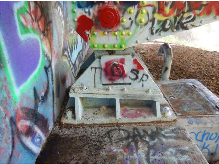
PHOTO 40 Condition Description Typical surface corrosion around masonry plate and 1-inch deep wear into bearing seat, looking east at west truss bearing Forward Abutment.
