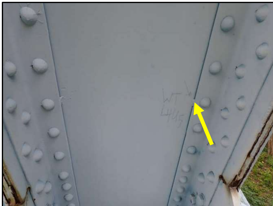
Photo 4 – Tack welds between angles and plates at ends of all diagonal members
