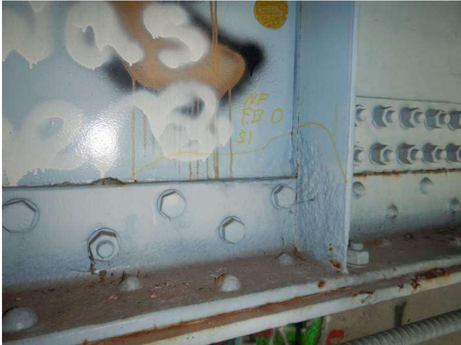
PHOTO 29 Condition Description Painted over pitting and section loss in bottom of web, typical, Floorbeam 0 shown, looking south.
