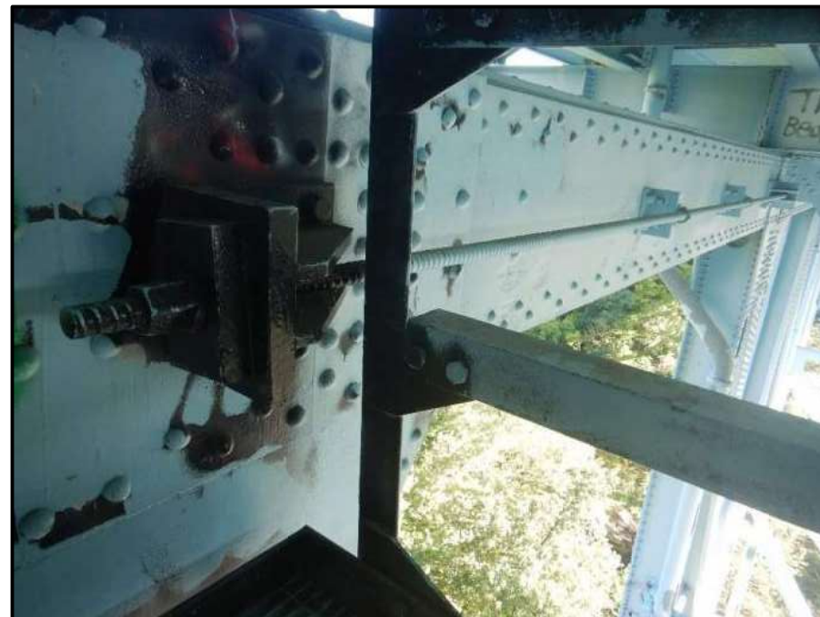
Photo 34 – Looking north along east face of west U7U8 at U7, span 2. Note: typical PT rod repair for upper chord.
