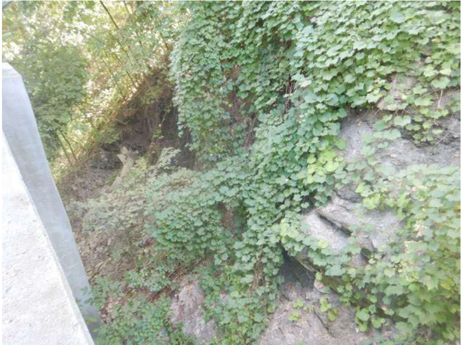
PHOTO 46 Condition Description South embankment is steep from erosion around Pier 1, looking southeast.
