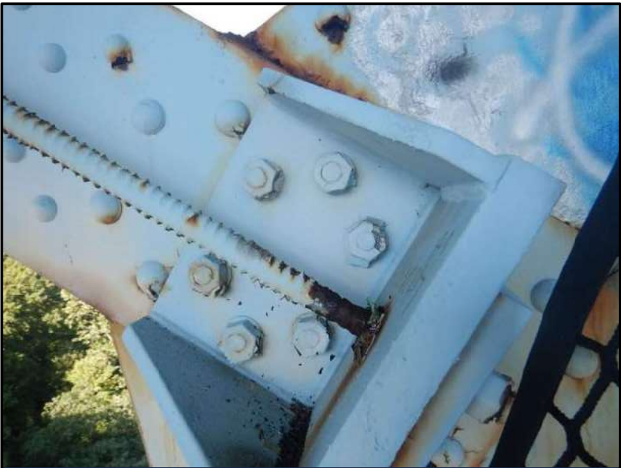
Photo 32 – Looking west at west U12L13 inboard PT rod, span 2. Note: rod exhibits up to 30% section loss, no change.
