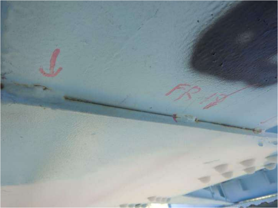
PHOTO 32 Condition Description Cracked bottom flange to upper lateral bracing gusset plate connection tack weld at Floorbeam 18, looking northwest.
