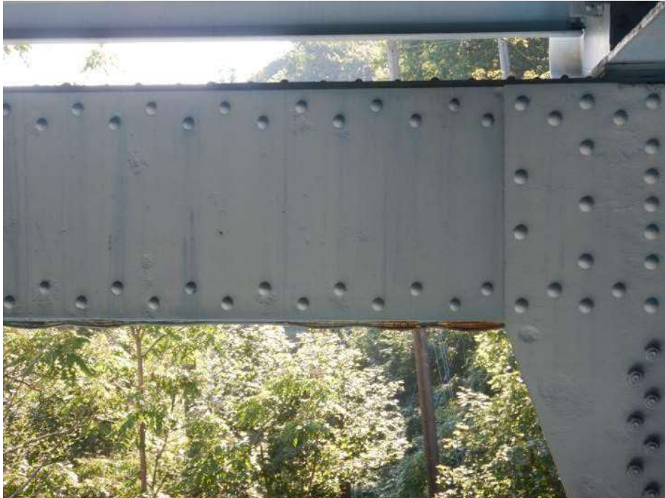
PHOTO 33 Condition Description Pack rust between bottom flange plate and fill plate up to 1-inch thick causing distortion, looking east at East U3U4 at U3.
