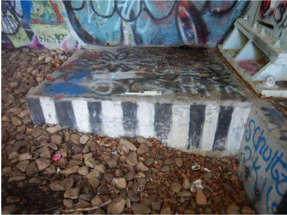
PHOTO 42 Condition Description 4-foot long x 1-foot tall delamination along top of breastwall, looking north at west end of Forward Abutment.
