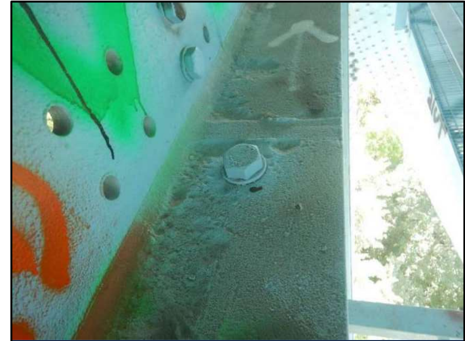
Photo 27 – Looking east along top of bottom flange of floorbeam 23, south face, span 3. Note: painted over section loss typically 3/16 inch deep.
