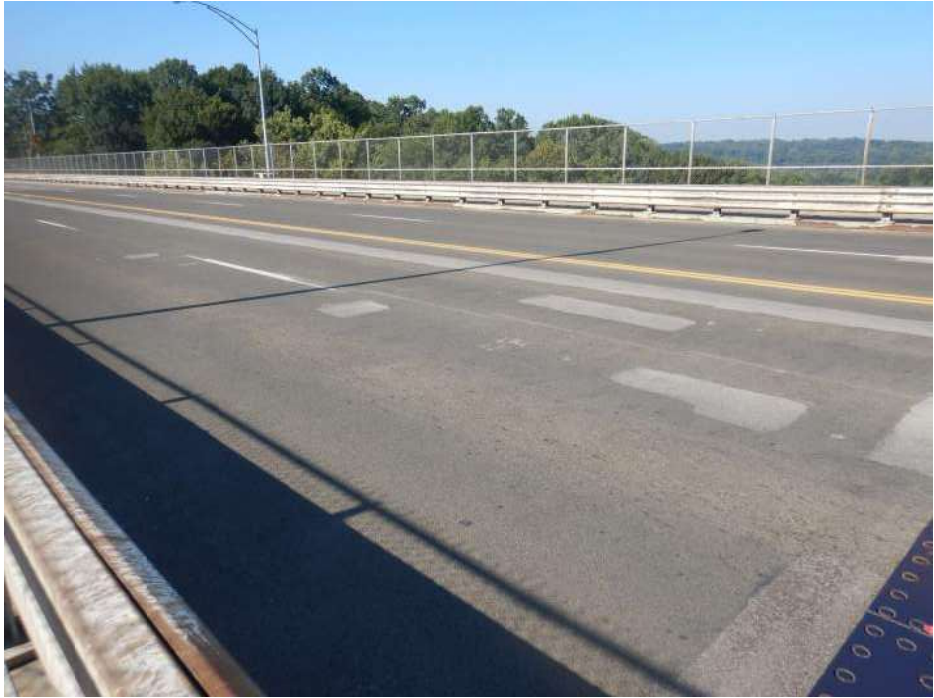
PHOTO 14 Condition Description Overall of deck wearing surface in Span 2, looking southwest. Note: Epoxy overlay and patches.
