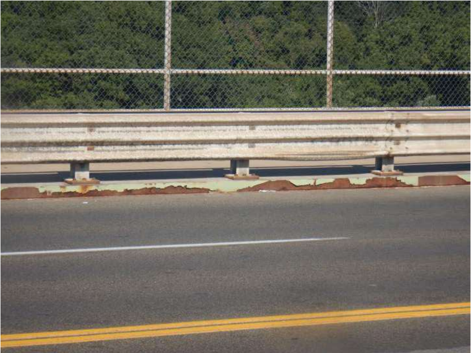
PHOTO 19 Condition Description Surface corrosion typical throughout longitudinal steel plate along curb, looking west.
