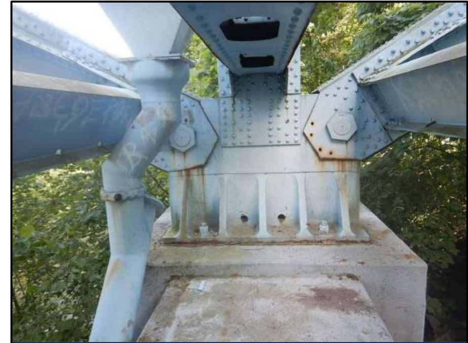
Photo 39 – Looking east at west face of east truss bearing at pier 1. Note: surface corrosion around masonry plate.
