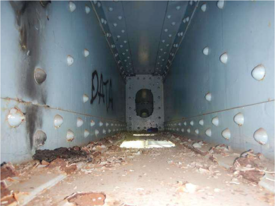
PHOTO 35 Condition Description Typical inside of lower chord with peeling paint and surface corrosion, heaviest along bottom flange, looking north.
