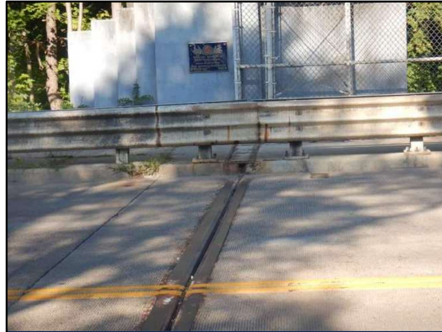
Photo 13 – Looking west at west end of rear abutment expansion joint at curb. Note: typical spall in curb at end of joint.
