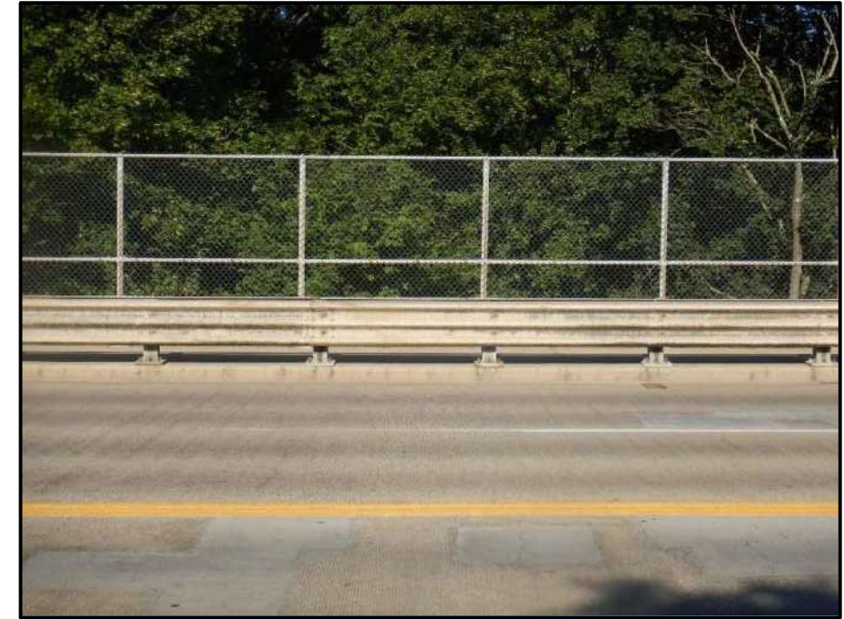
Photo 3 – Looking west at the west sidewalk and railings. Note: typical minor corrosion throughout thrie-beam railing.
