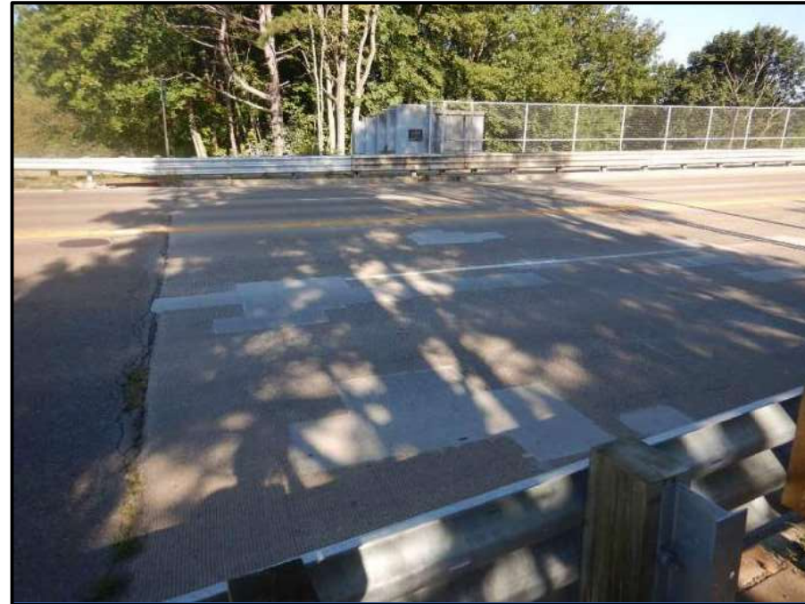
Photo 53 – Looking northwest at rear approach slab. Note: sound patches throughout northbound lanes.
