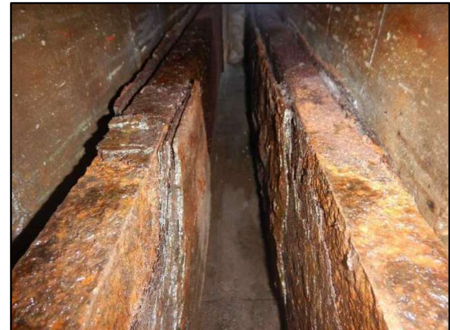
Photo 40 – Looking north at west truss eye bar tie down anchorage at forward abutment. Note: 1/16-inch deep pitting and laminating corrosion on eye bars.
