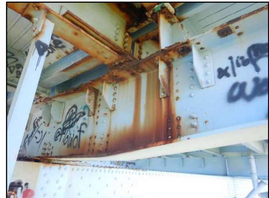
Photo 28 – Looking southeast at west end of floorbeam 17, north face, span 2. Note: heavy corrosion and rust staining.
