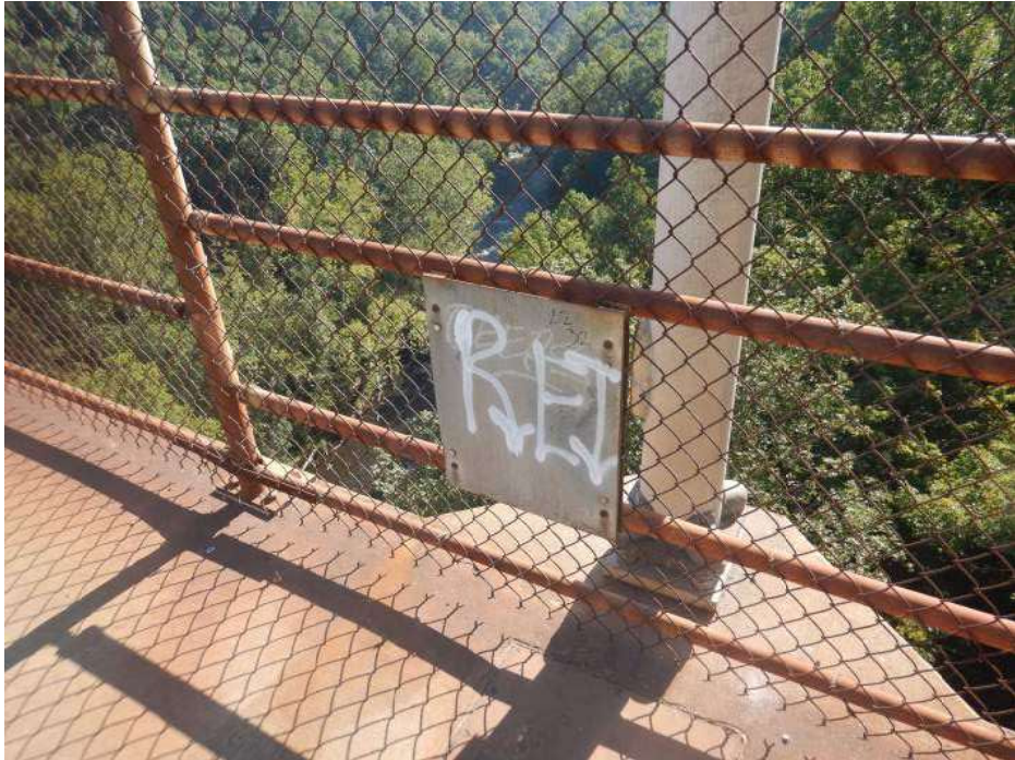
PHOTO 17 Condition Description Typical steel plate repair to east pedestrian fencing, looking east.
