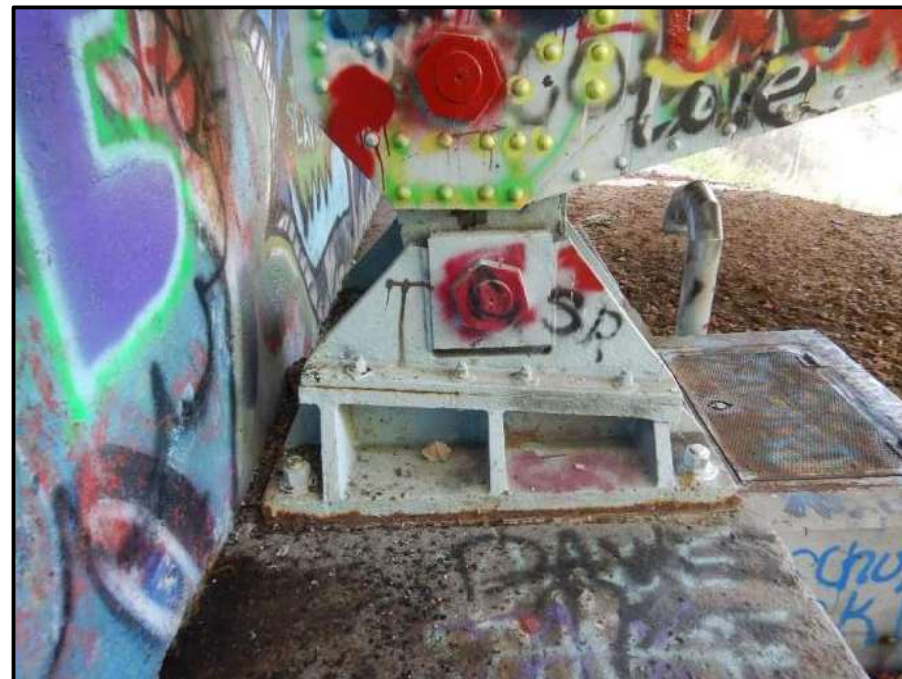
Photo 38 – Looking east at west truss bearing at forward abutment. Note: surface corrosion around edges of masonry plate with 1-inch deep wear into bearing seat.
