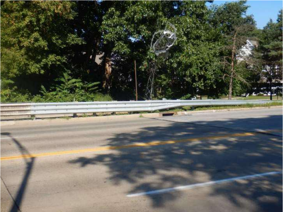
PHOTO 49 Condition Description New approach guardrail, typical at all four corners of bridge, looking northwest at northwest approach.
