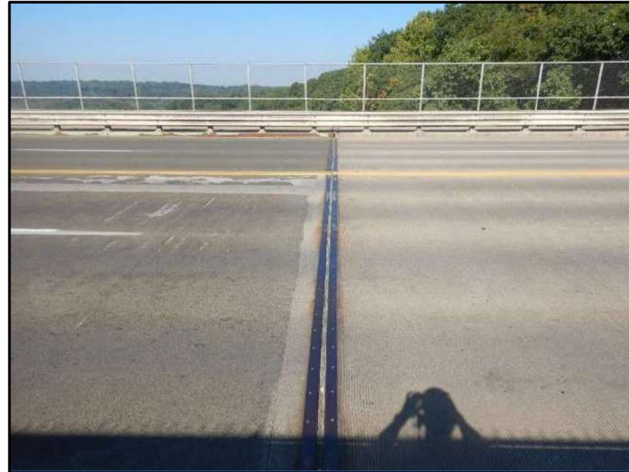
Photo 21 – Looking west at pier 2 strip seal joint. Note: minor debris in joint.
