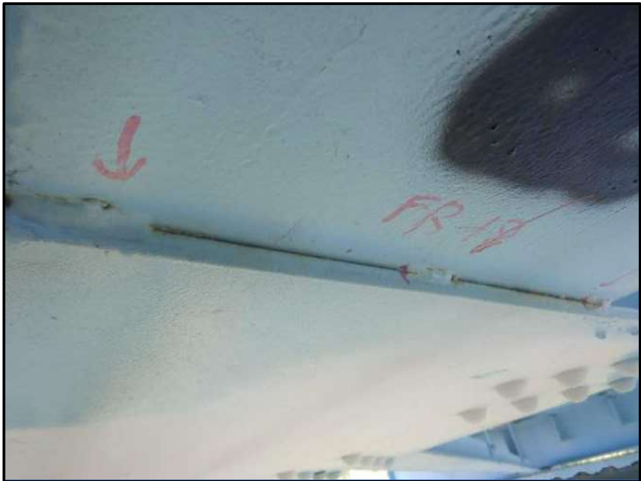
Photo 29 – Looking northwest floorbeam 18 bottom flange connection to lower lateral bracing connection plate, span 2. Note: cracked tack welds.
