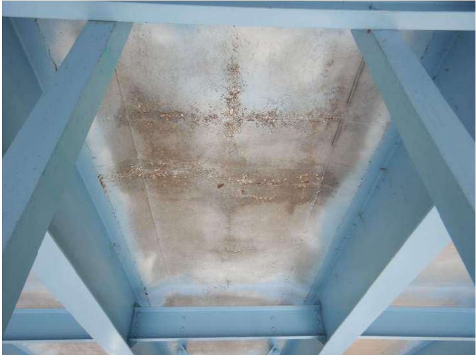
PHOTO 21 Condition Description Isolated transverse cracks with minor efflorescence in Span 1 deck soffit, looking south.
