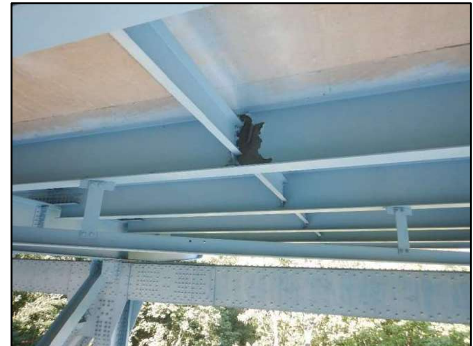
Photo 24 – Looking west at east face of stringer 5 between floorbeams 5 and 6, span 1. Note: 2 square feet of peeling paint exposing primer.
