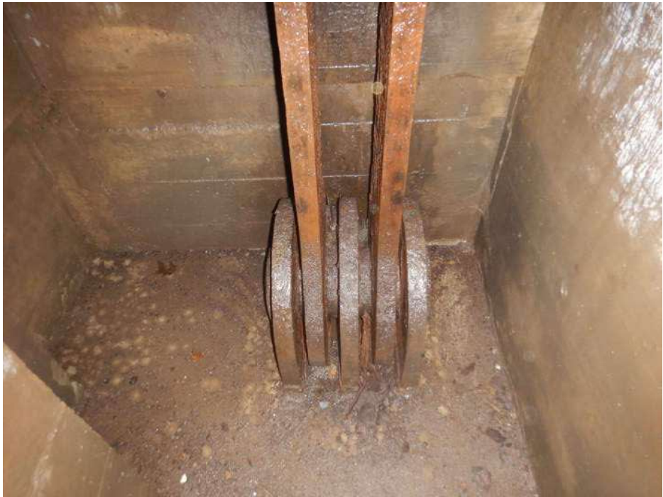
PHOTO 38 Condition Description Eyebar tie-down anchorage with 1/16-inch deep pitting and laminating corrosion at Forward Abutment, looking north.
