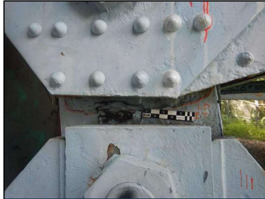
Photo 37 – Looking west at east truss bearing at rear abutment, east face. Note: 3/16-inch deep painted over section loss to exterior of outboard pin plate, no change.
