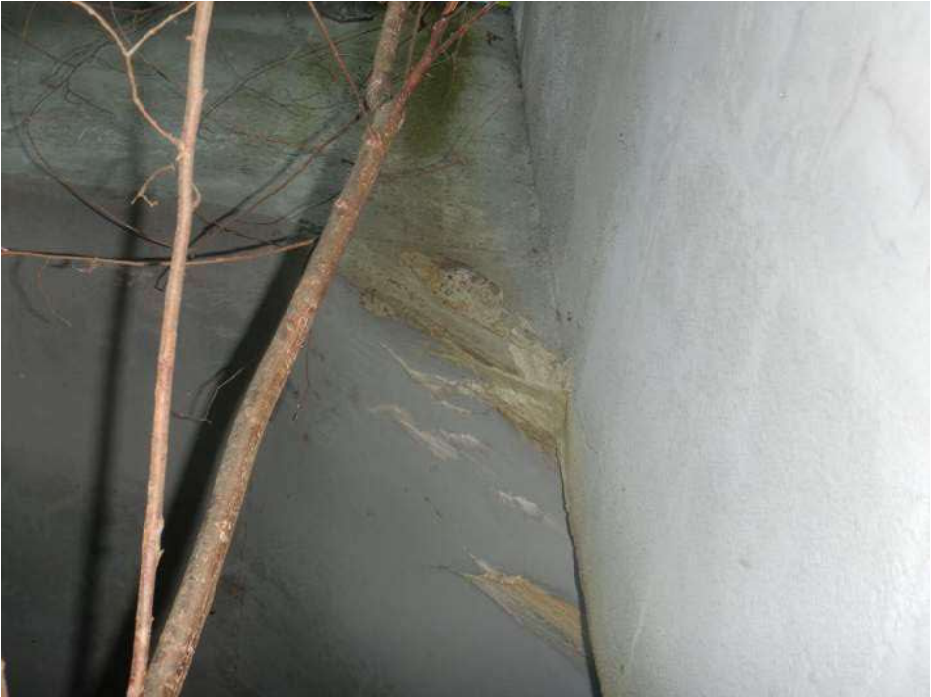
PHOTO 43 Condition Description 2-foot long x 1-foot wide x 1-inch deep spall with adjacent efflorescence in north face of west end of Pier cap 1, looking south.
