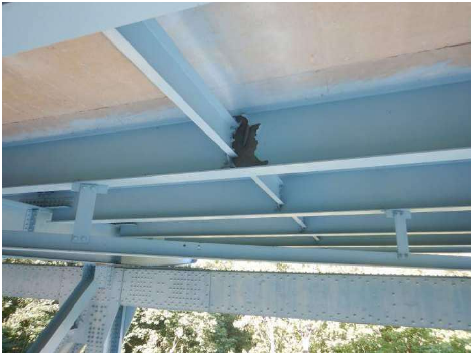
PHOTO 26 Condition Description 2-square-feet of peeling paint on Stringer 5 between Floorbeams 5 and 6, Span 1, looking west.
