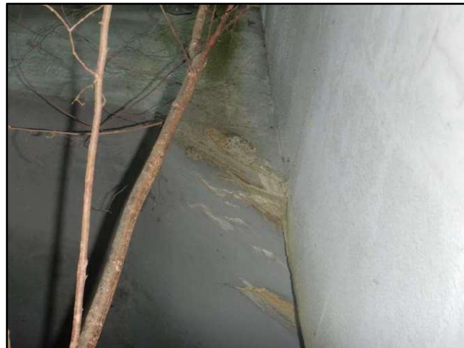
Photo 46 – Looking south at north face of pier 1 cap at column 1. Note: 2-foot long x 1-foot wide x 1-inch deep spall with adjacent efflorescence.
