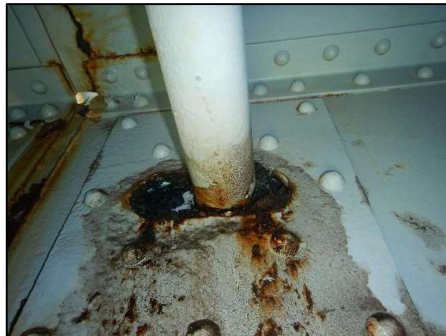
Photo 42 – Looking east at interior of pin at west U13, span 2. Note: painted over section loss and active corrosion in pin plate.
