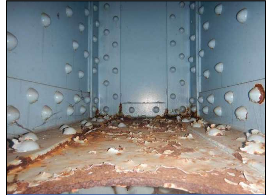
Photo 35 – Looking south at west L0L1 at the rear abutment, span 1. Note: heavy corrosion and peeling paint along bottom flange plate interior.
