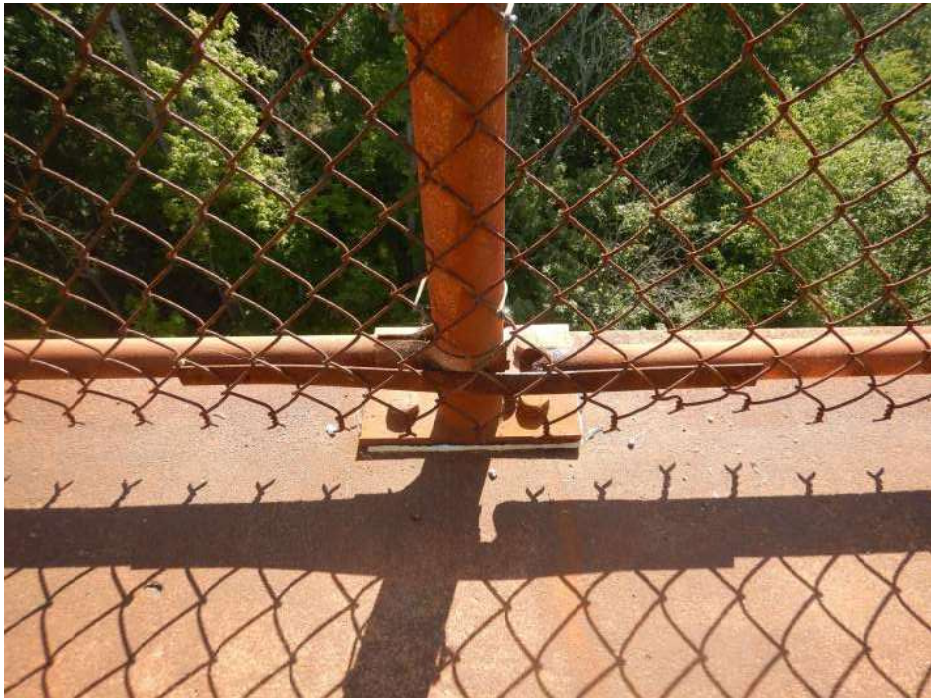
PHOTO 18 Condition Description Repair to corroded horizontal piping for east pedestrian fence, typical, looking east.
