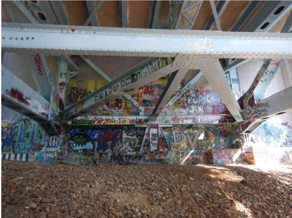
PHOTO 41 Condition Description Overall of Forward Abutment, looking north. Note: Backwall and breastwall covered with graffiti.
