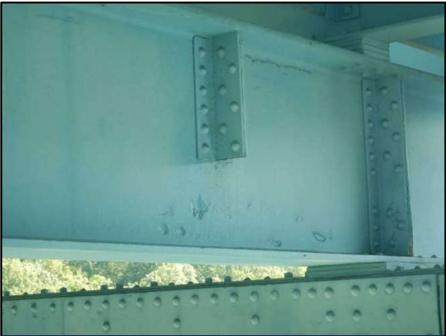
Photo 31 – Looking northeast at south face of floorbeam 14 web under stringers 7 and 8, span 2. Note: multiple gouges in web most likely from construction.
