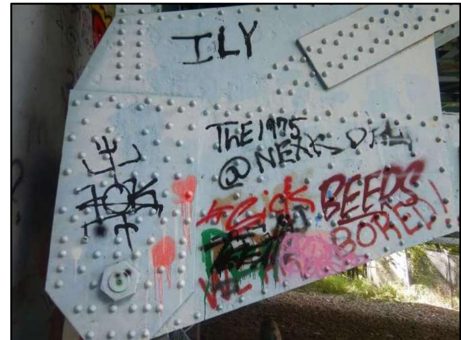
Photo 36 – Looking west at east L0 outboard gusset plate at rear abutment. Note: graffiti and isolated areas of painted over section loss.
