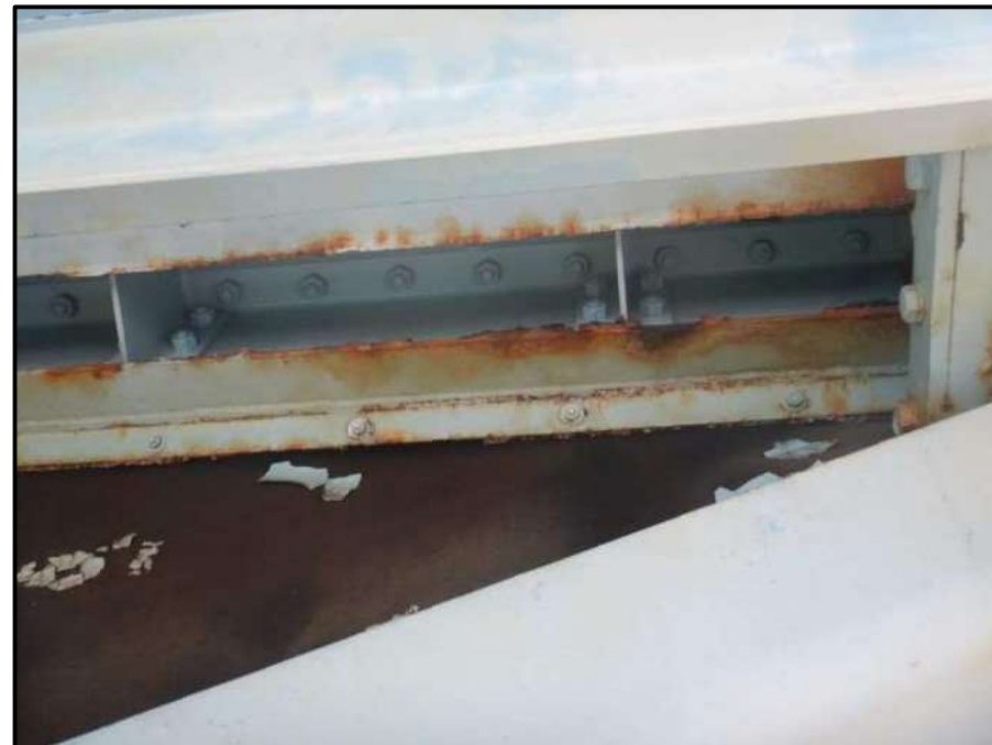
Photo 22 – Looking north at underside of top flange of floorbeam 13 below finger joint. Note: corrosion to floorbeam from previous leakage. Neoprene flashing sheet in place to direct water.
