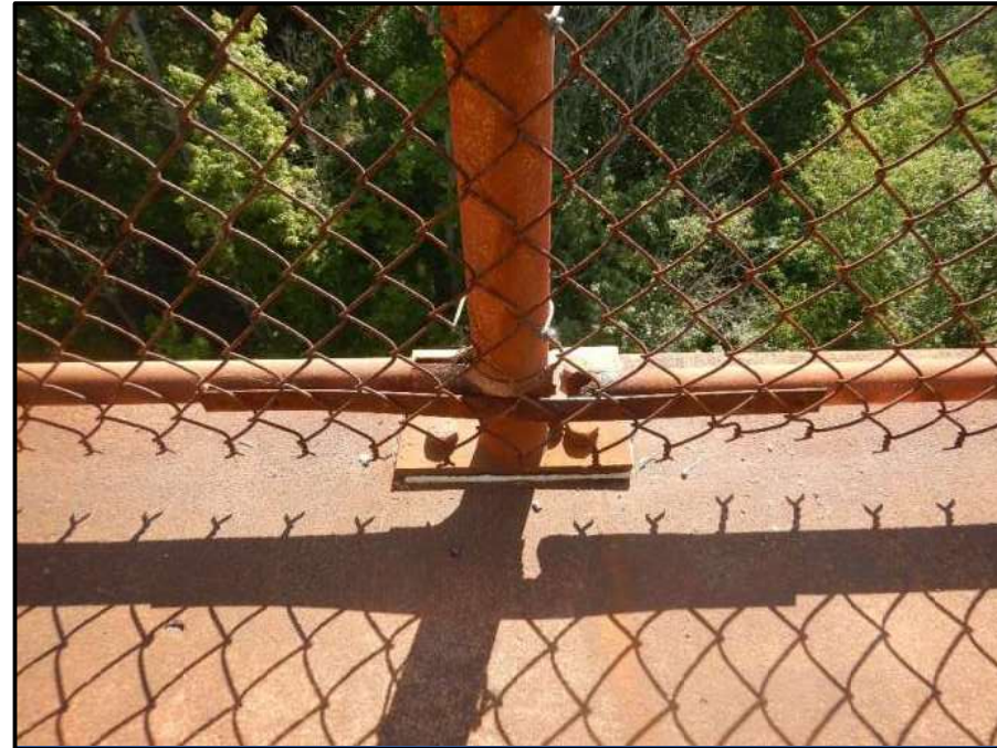
Photo 5 – Looking east at east pedestrian fence base connection in span 3. Note: steel longitudinal retainer plate repair due to previous heavy corrosion.
