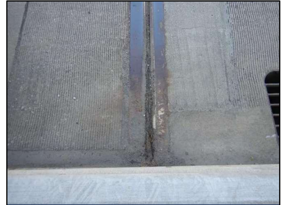
Photo 23 – Looking west at east end of rear abutment strip seal joint. Note: typical corrosion and minor section loss to joint armor.
