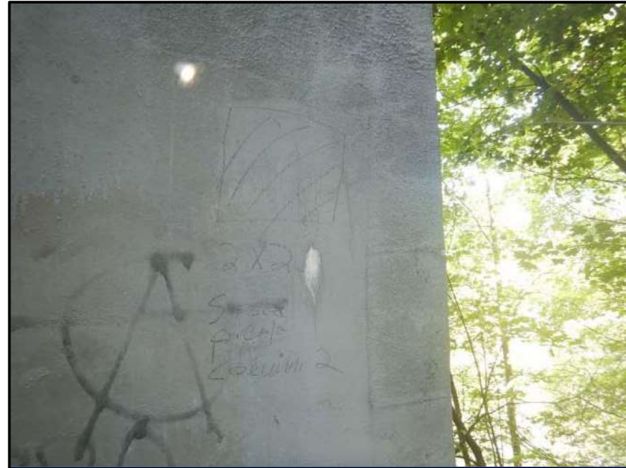
Photo 45 – Looking north at south face of column 2, pier 1 approximately 7 feet above the ground. Note: 2-foot x 2-foot delamination.
