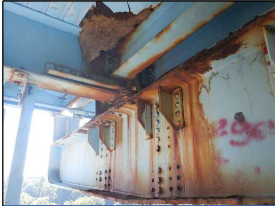
Photo 25 – Looking southeast at stringer 11 connection to north face of floorbeam 17, span 2. Note: heavy corrosion and pack rust under stringer bearing.
