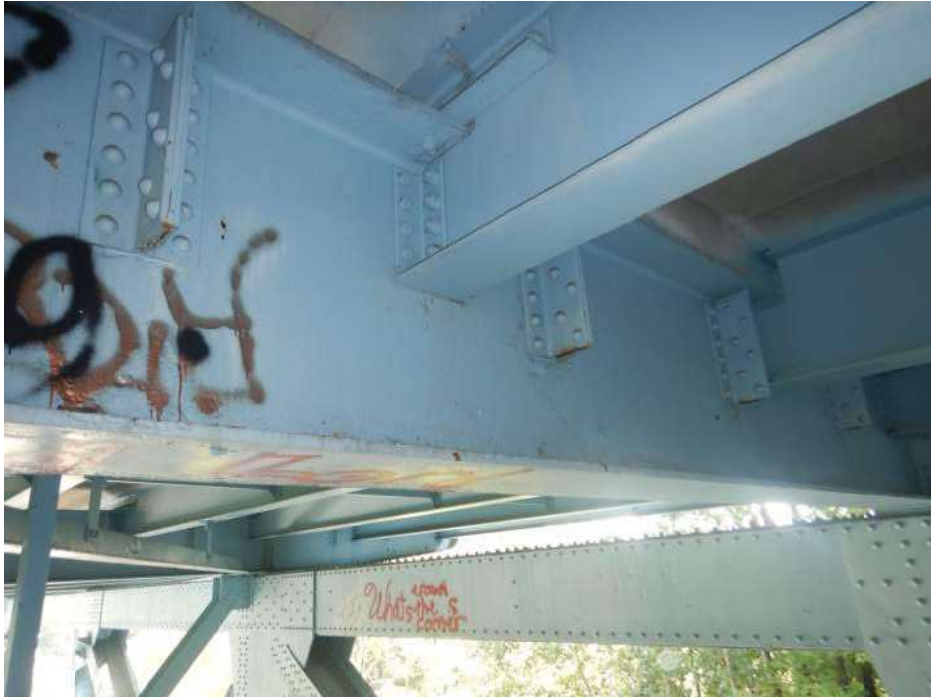
PHOTO 30 Condition Description Abandoned stringer attachment angles, typical, Floorbeam 1 shown, looking northeast.
