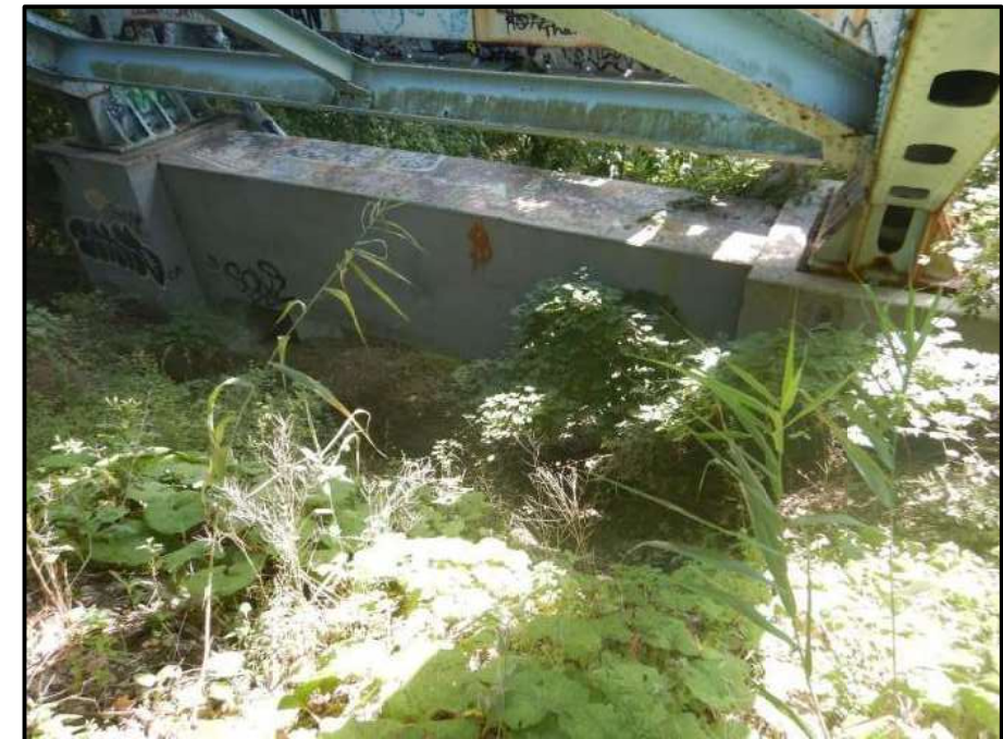
Photo 47 – Looking at pier 2 at heavy vegetation growth around cap and columns.
