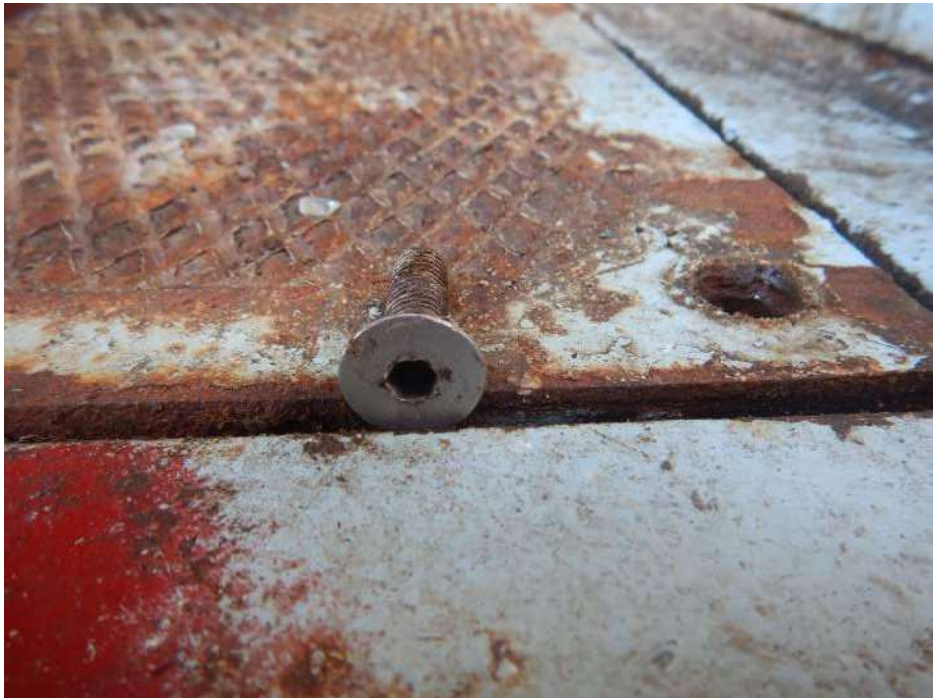
PHOTO 10 Condition Description Stripped hex head screws for hatches to eyebar linkages at abutments looking west.
