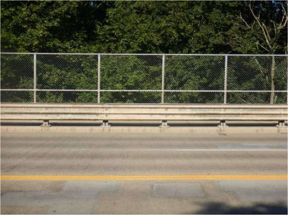
PHOTO 16 Condition Description Typical bridge railing with minor corrosion throughout, west railing shown, looking west.
