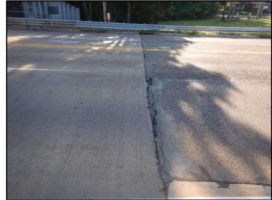
Photo 55 – Looking east along approach slab to asphalt roadway transition at rear approach. Note: edge spalling along asphalt.
