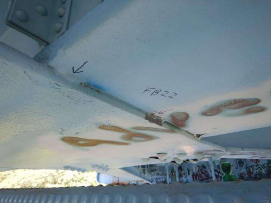
PHOTO 31 Condition Description Typical upper lateral bracing gusset plate connection to floorbeam tack welds, looking northwest.
