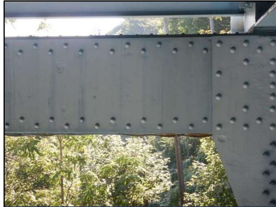
Photo 33 – Looking east at east U3U4 at U3, west face, span 1. Note: typical painted over section loss to web of upper chord. Pack rust up to 1 inch thick between bottom plate and bottom of web.
