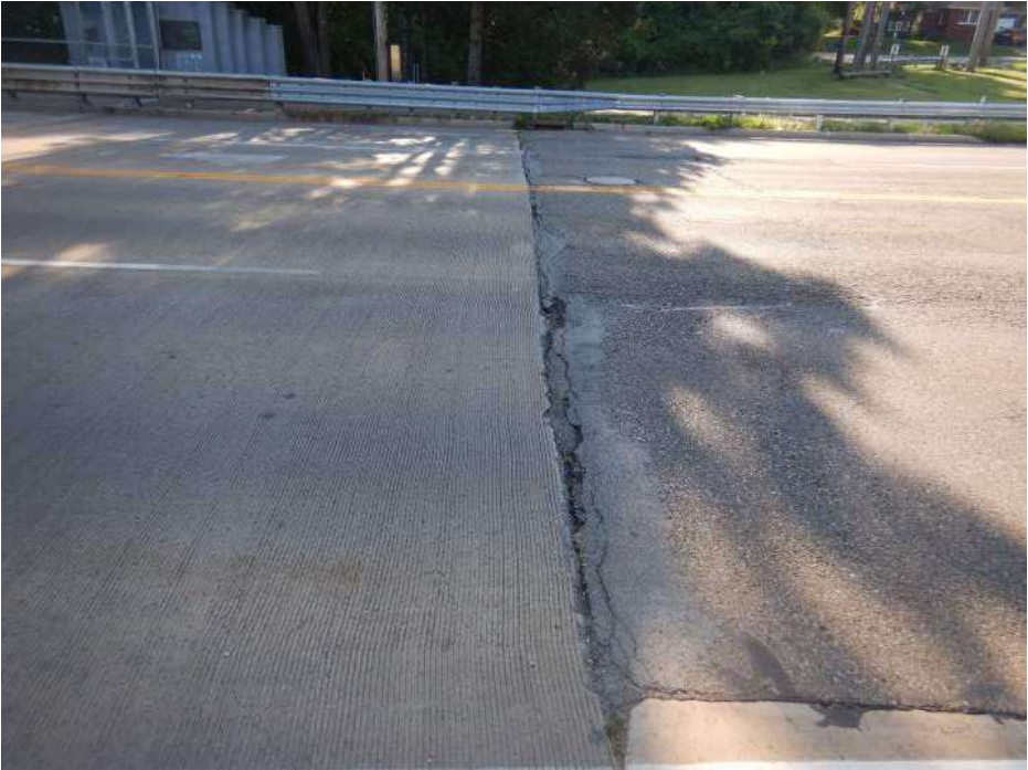
PHOTO 47 Condition Description Spalling along edge of asphalt roadway at Rear Approach slab with failing patches, looking east.
