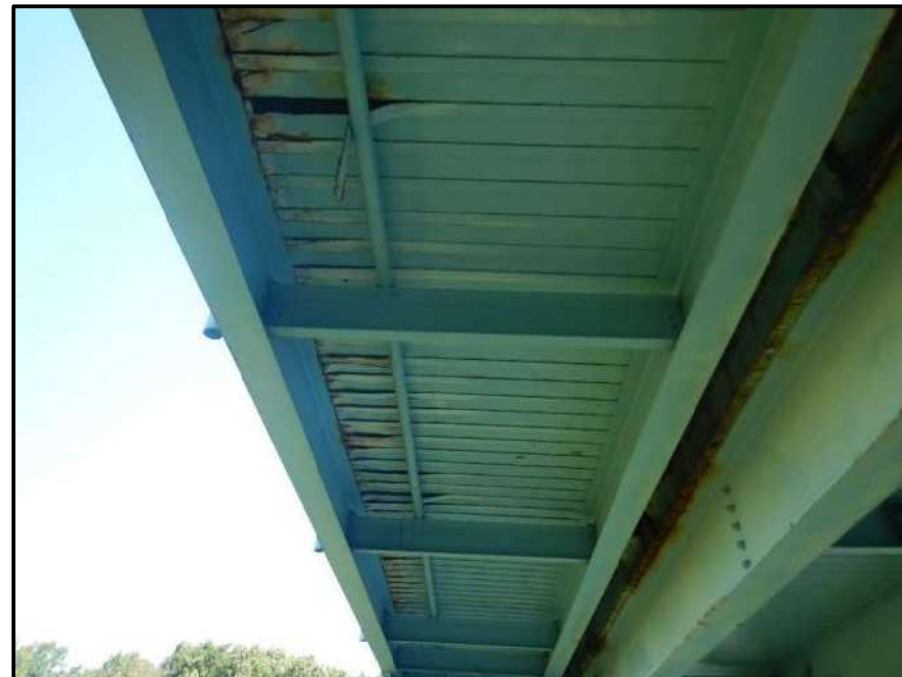
Photo 14 – Looking north under west sidewalk at steel SIP forms, span 2. Note: heavy corrosion and failing paint throughout.
