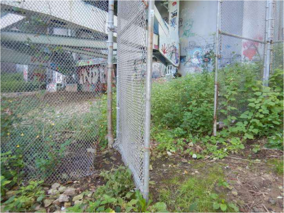
PHOTO 7 Condition Description Hole in chain link fence by gate at southwest corner, looking southeast.
