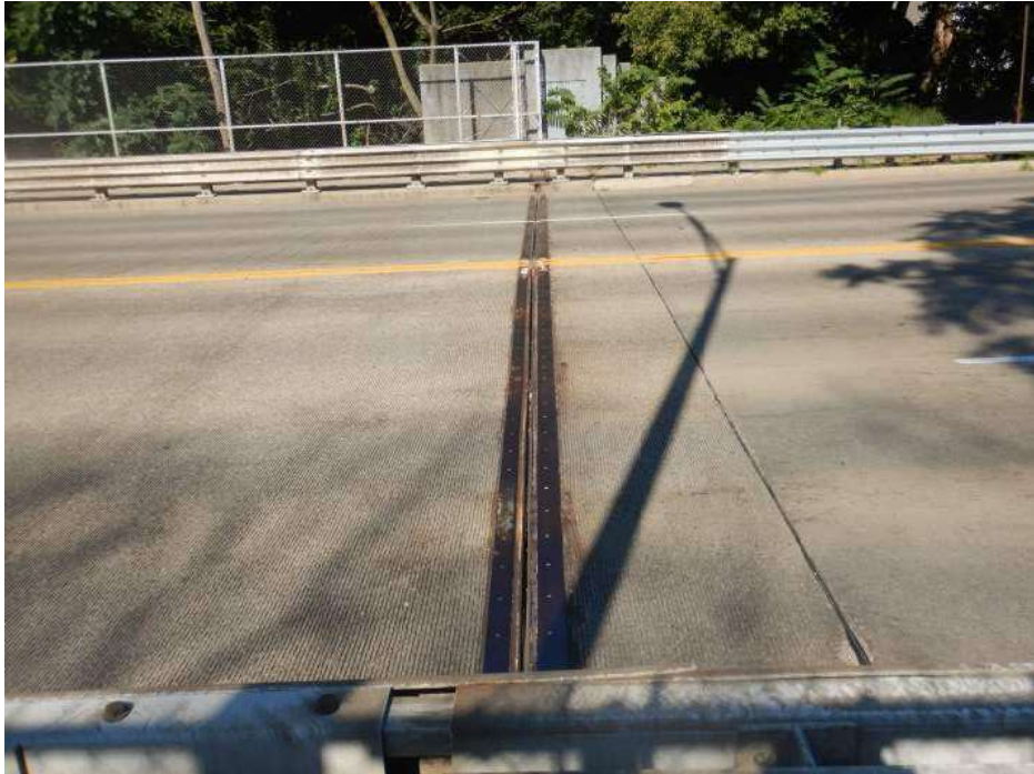
PHOTO 25 Condition Description Strip seal at Forward Abutment, looking west.
