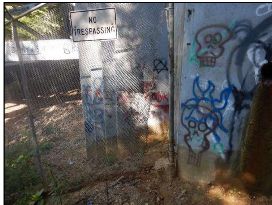
Photo 10 – Looking west at hole in the fence at the west end of the forward abutment.
