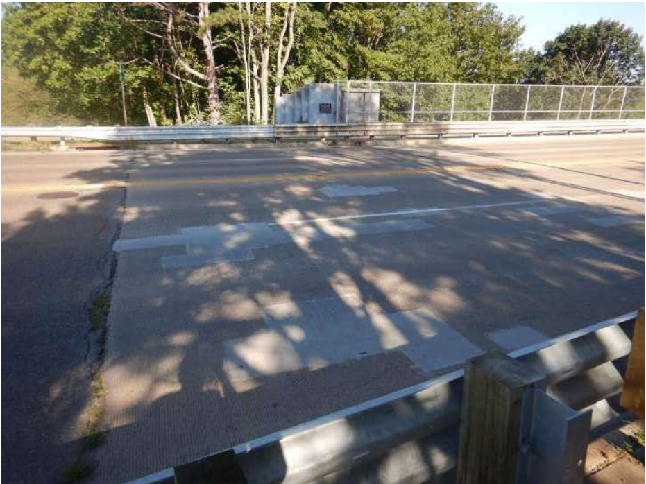
PHOTO 48 Condition Description Sound patches in NB lanes at Rear Approach, looking northwest.
