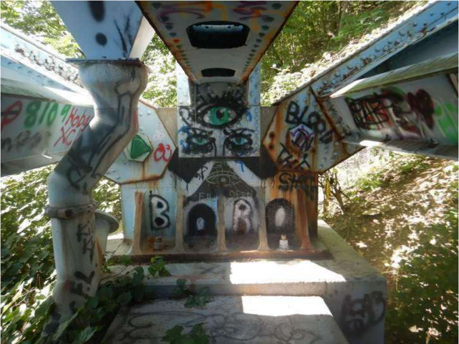
PHOTO 39 Condition Description Fixed bearing, typical, looking west at west truss bearing at Pier 2.
