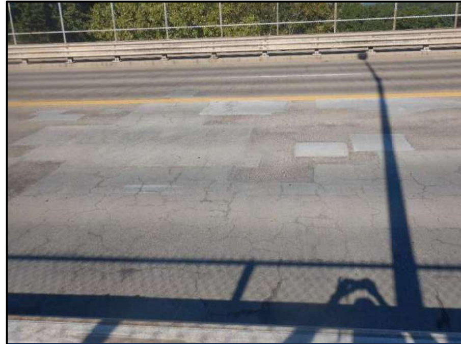
Photo 17 – Looking west at northbound lanes of bridge wearing surface in span 1. Note: cracking in patches throughout.
