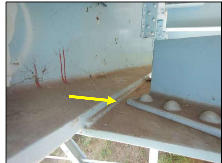
Photo 6 – Fillet weld along bottom flange of floorbeam at lateral bracing center connection plate
