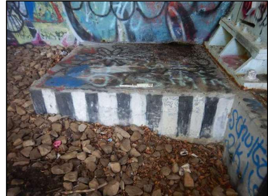
Photo 43 – Looking north at west end of forward abutment along top of breastwall. Note: 4-foot long x 1-foot tall delamination.
