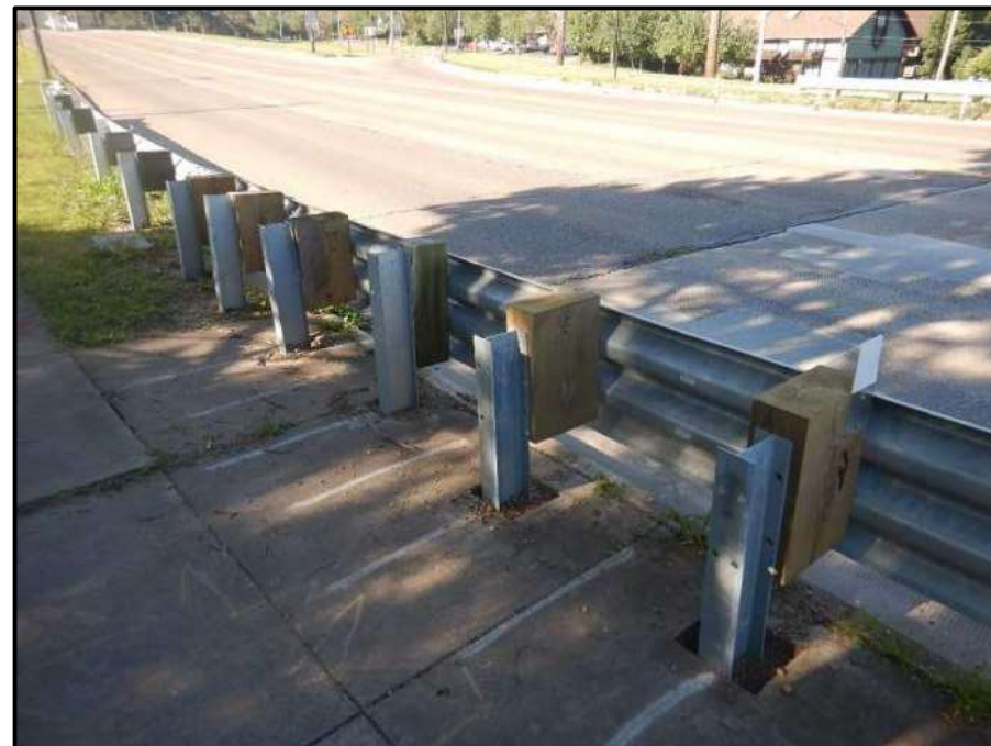
Photo 6 – Looking southwest at newly installed approach guardrail along east side of the rear approach.
