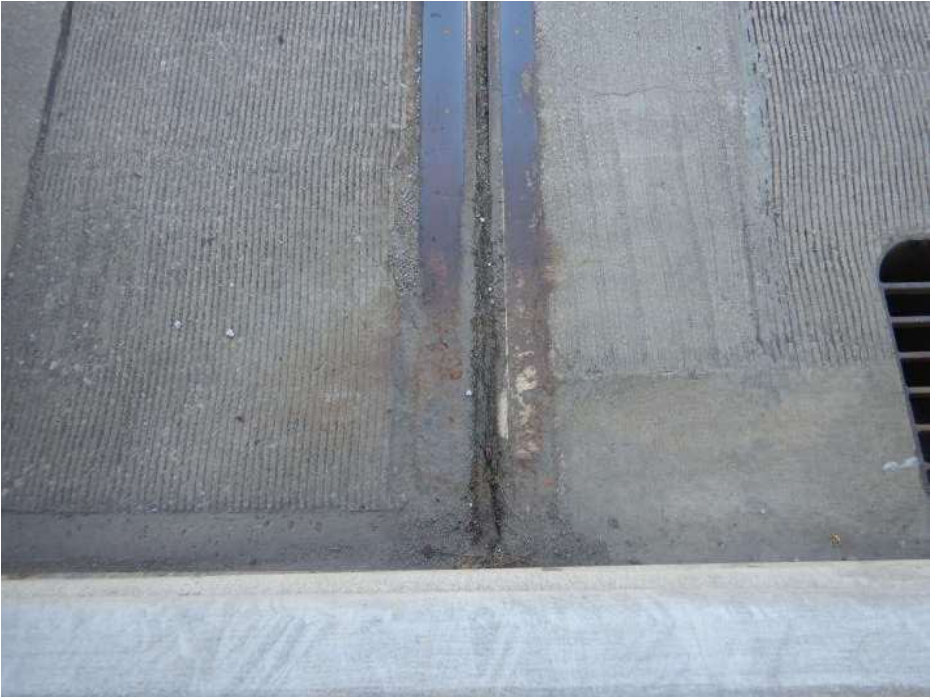
PHOTO 23 Condition Description Surface corrosion and minor section loss to joint armor from debris, Rear Abutment joint at east end, looking west.
