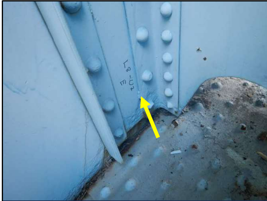
Photo 3 – Tack welds connecting angles to vertical plates on exterior of upper & lower chord box members, near the ends of the member.
