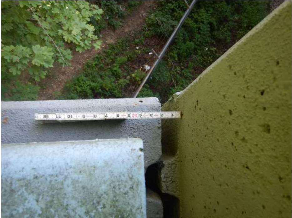
PHOTO 45 Condition Description Southwest wingwall has rotated away from Rear Abutment, 1 3/4 inches measured at top, looking north.
