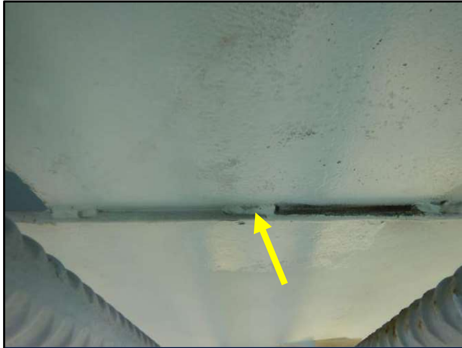
Photo 7 – Tack welds across bottom of bottom flange of floorbeam at lateral bracing connection plates.
