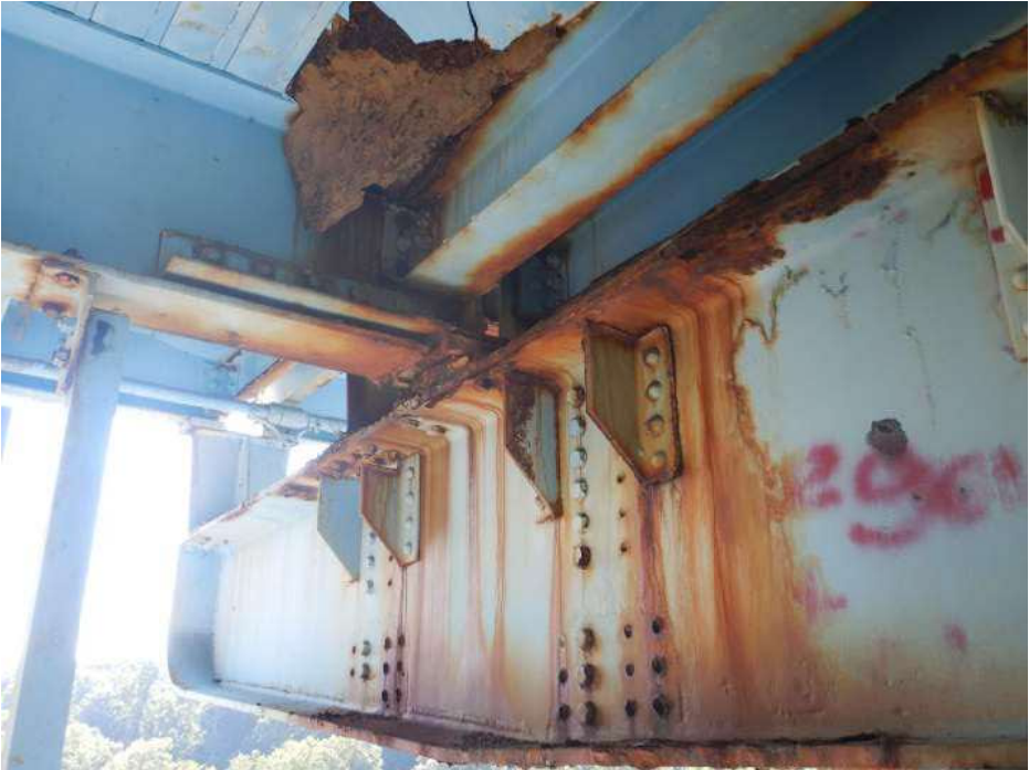
PHOTO 27 Condition Description Heavy corrosion and pack rust under Stringer 11 bearing over Floorbeam 11, Span 2, looking southeast.
