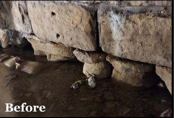
Above: Maintenance on The Akron Peninsula Rd Bridge (BST 10-1010) shows photos Before, During, and After repairs made to the wing walls.
