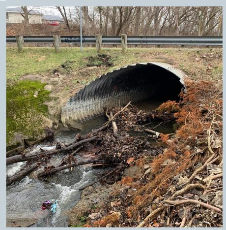
Shadybrook Rd. over Springfield Lake Outlet. Inspectors noted debris at end of pipe. SCE Crews removed.
