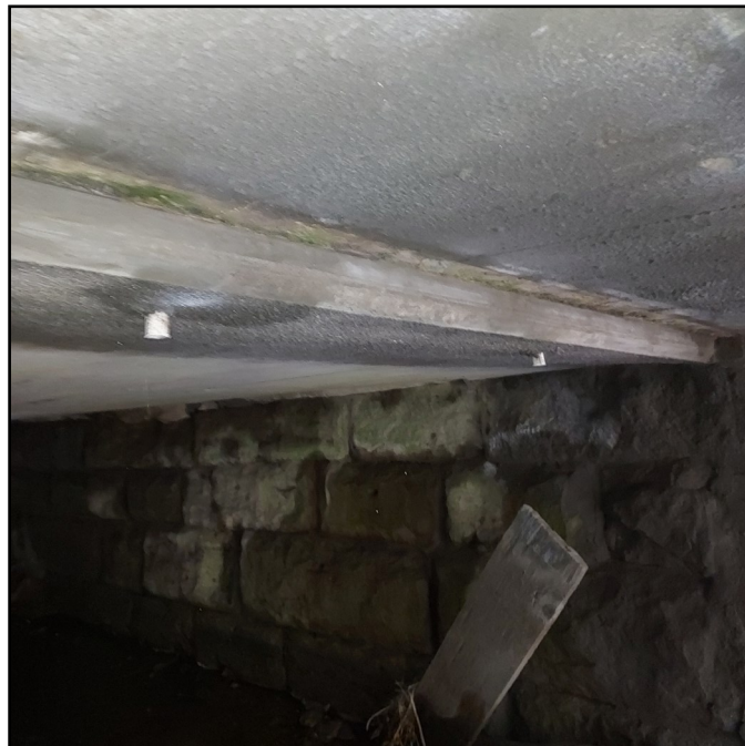
Work completed under Shaw Rd Bridge
