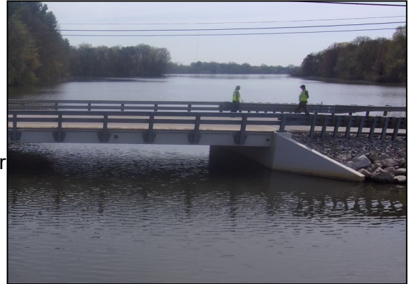
Annual Inspection—Cleveland Massillon Rd Bridge over Wolf Creek COP-017-1141
