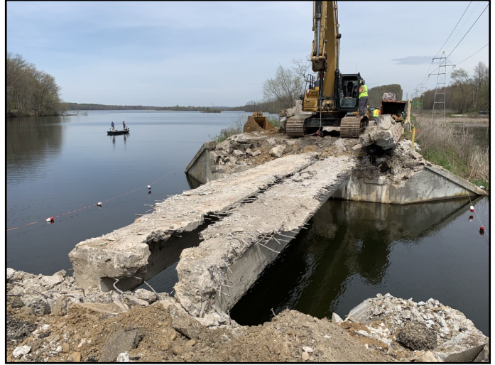
Christman Rd Bridge Demolition
