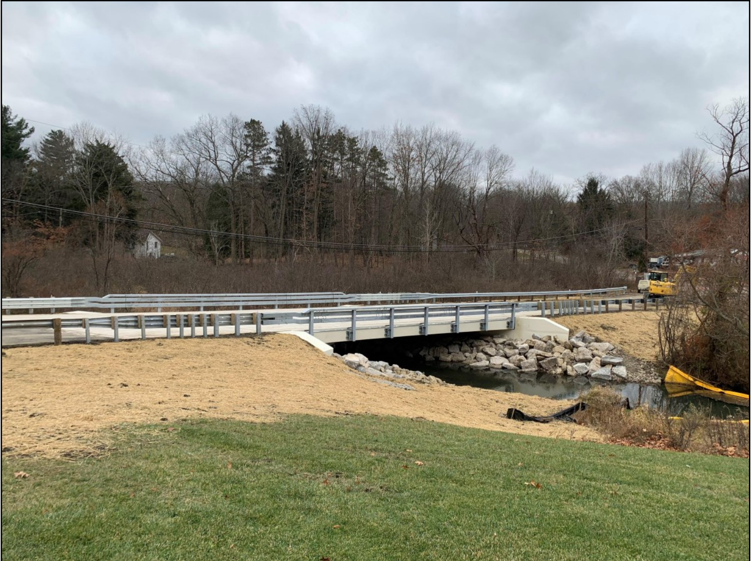
Pressler Road Bridge Replacement
