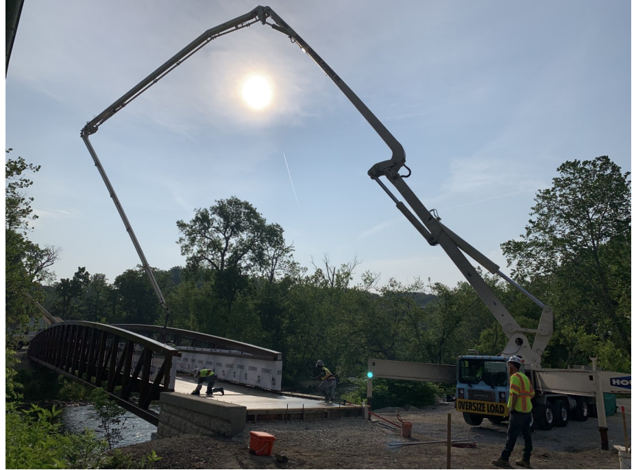
Construction of the Cuyahoga Valley Pedestrian Bridge
