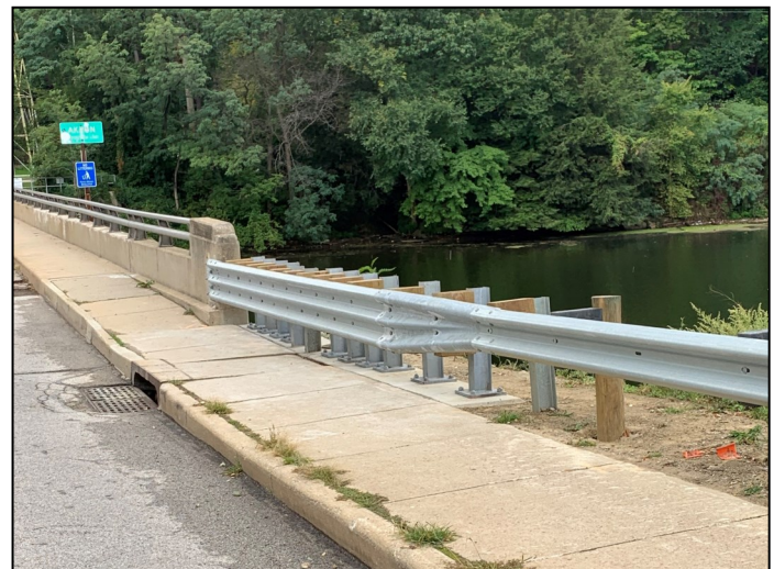
Front St Bridge over the Cuyahoga River AKR-059-0275
