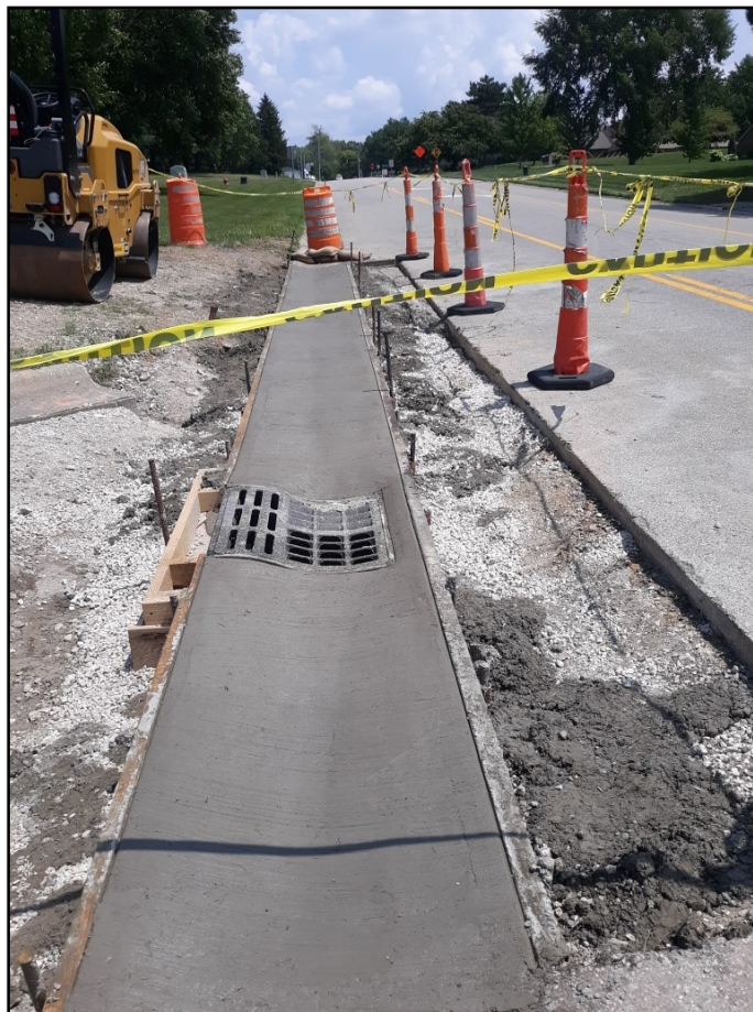
Basin Repair on Springside Dr
