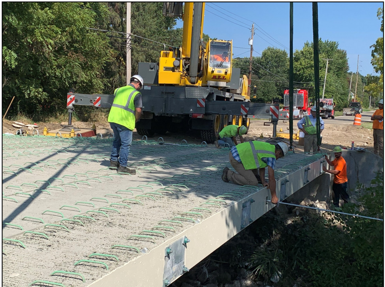
South Main Street Bridge over Nimisila Creek
