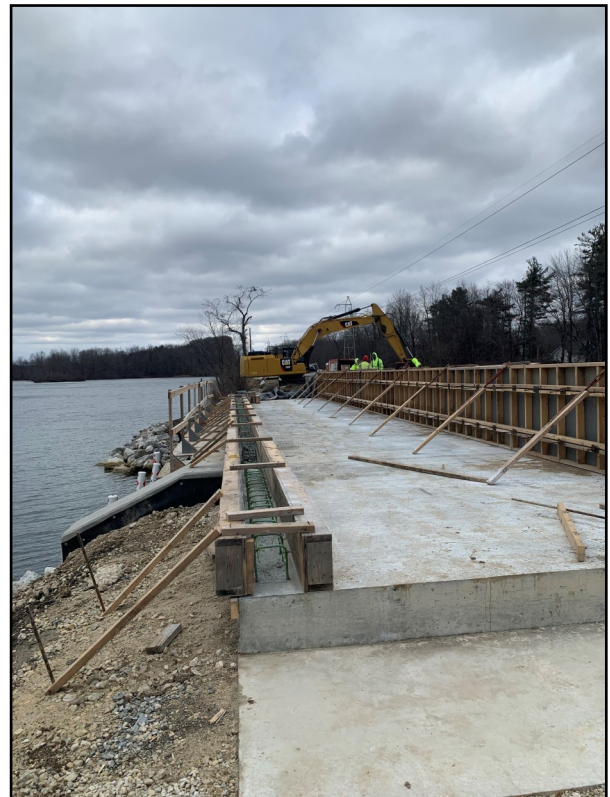
Christman Rd Bridge replacement
