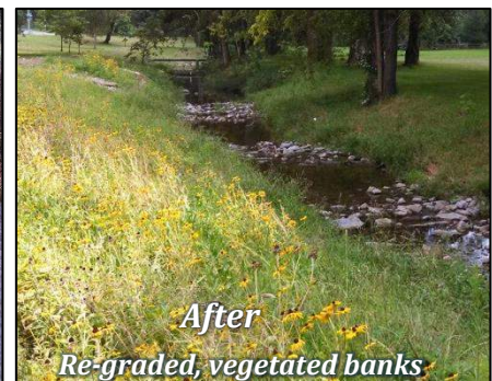
Stabilized bank with re-graded 4:1 slopes and riparian vegetation
