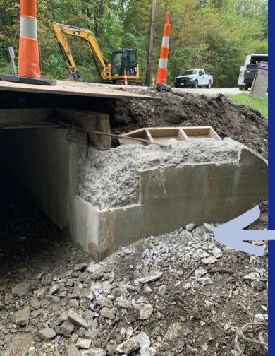
On Revere Road the Bridge Crew is currently repairing a culvert using gunite and redi-mix. The project which is currently ongoing is being done to repair deterioration of a culvert that Road Maintenance Manager Kurt Koerber said was more than likely last replaced in the 1930s.
