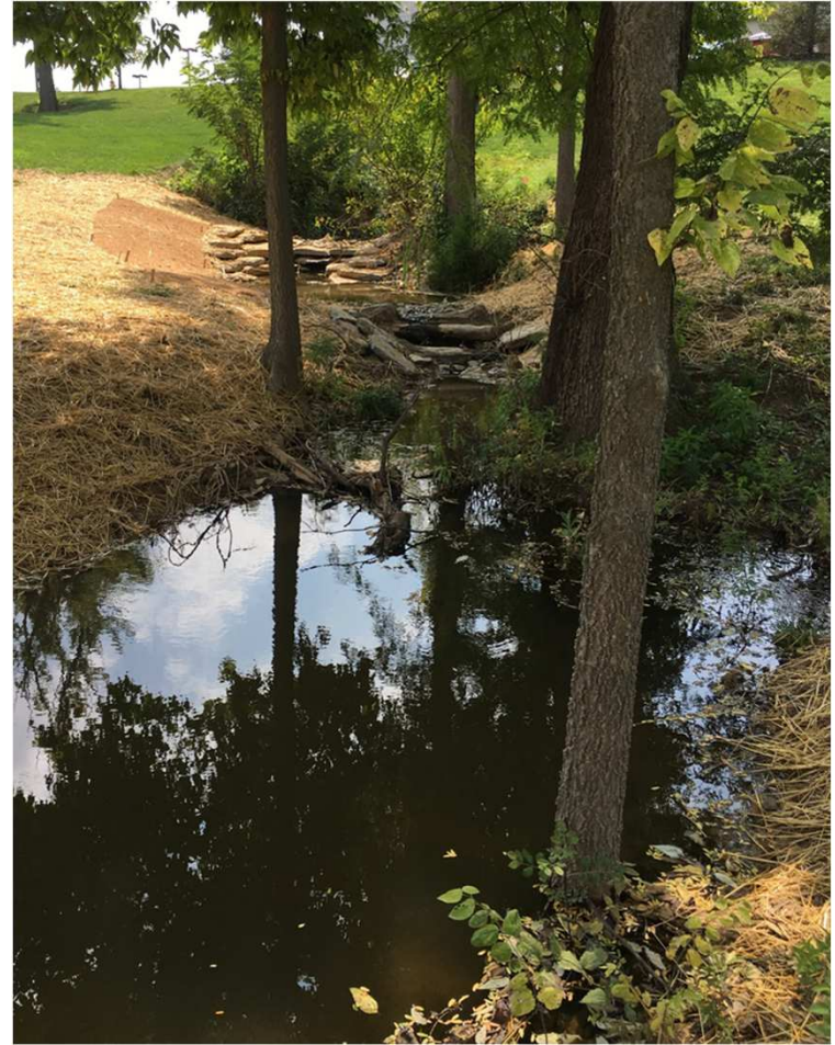
Armoring and step-pools stabilize the stream.
