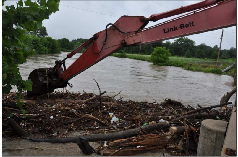
Debris and flood waters threatening to wash out the Bolanz Bridge over the Cuyahoga in July 2011. Photo credit: Robert Eller
