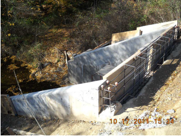
Cleveland Massillon Road Bridge Wing Wall Reconstruction
