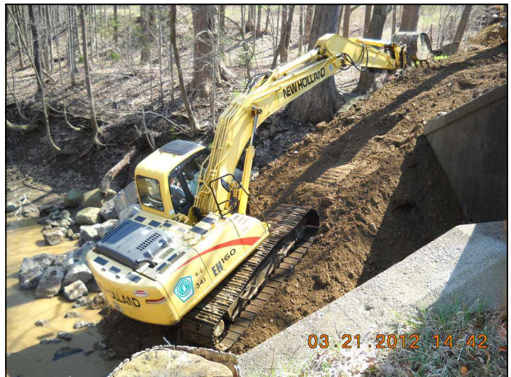
North Fork erosion project
