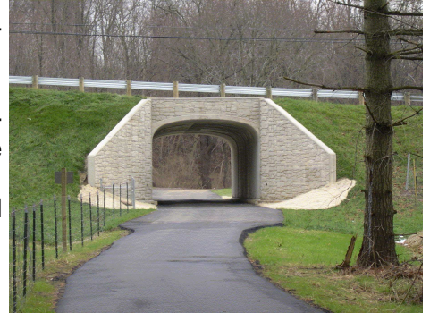
Bath Nature Preserve Underpass
