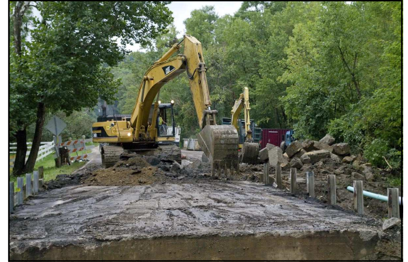
Northampton Road Bridge Replacement
