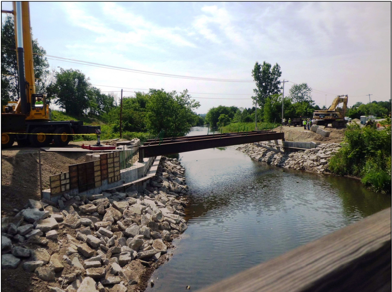
Van Buren Road Bridge over the Tuscarawas River Replacement Project
