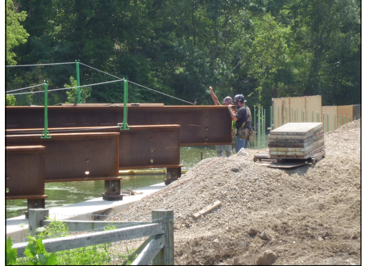
Beam setting on the Van Buren Road Bridge over the Tusc
