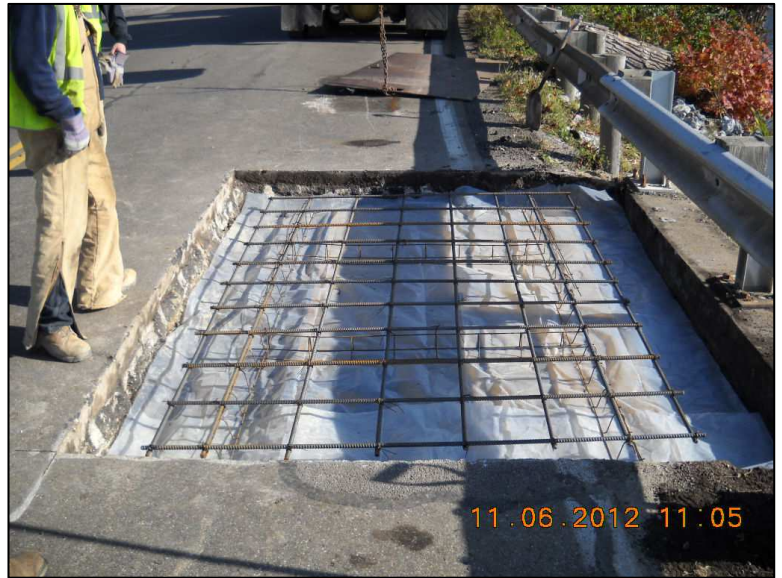
Portage Lakes Drive Culvert Repair
