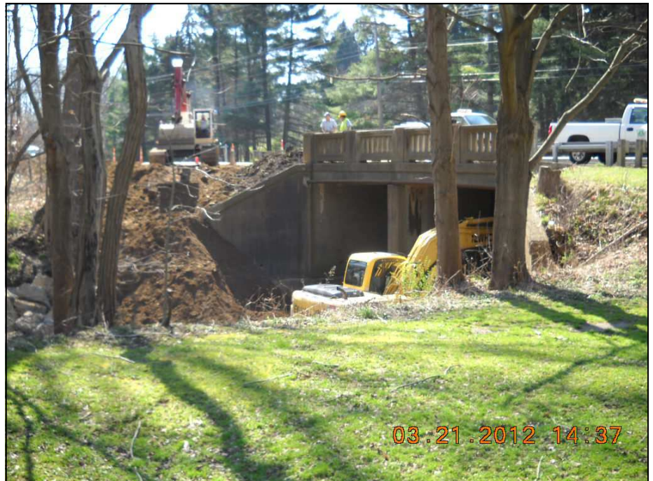
North Fork erosion project
