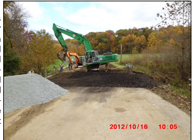
Akron Peninsula Road Improvements
