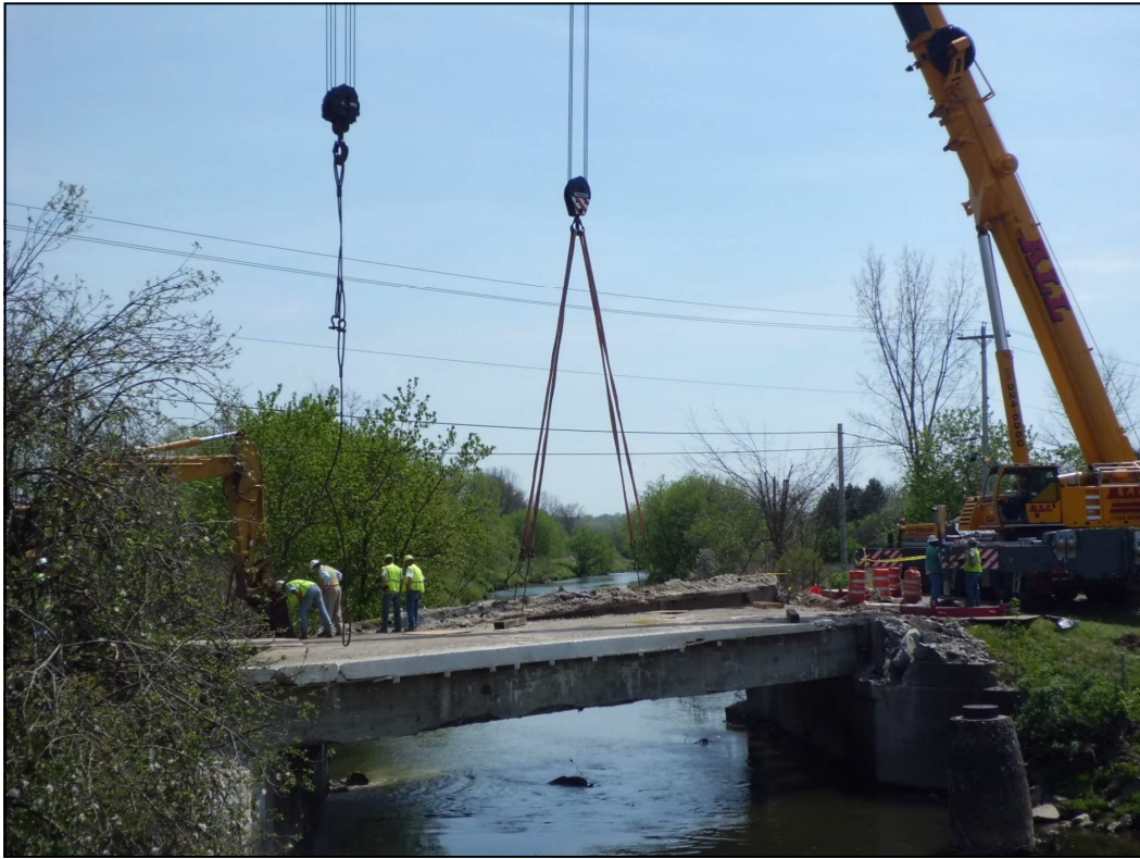
Van Buren Road Bridge Replacement Beam setting
