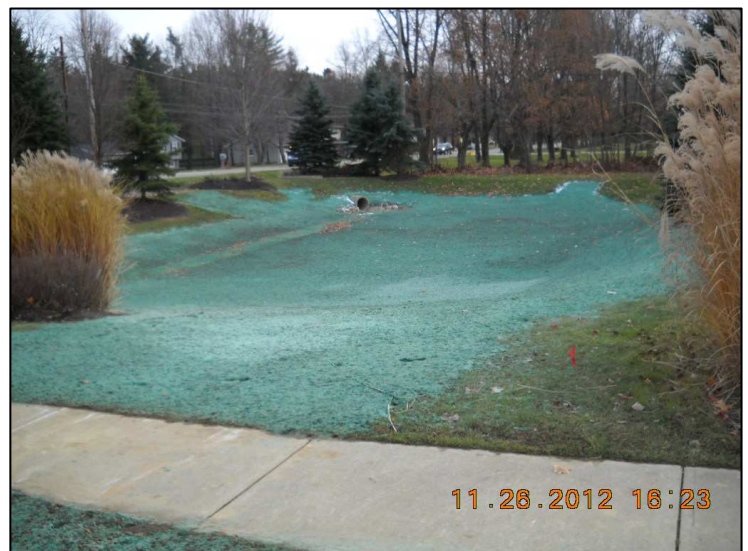
Hillside Allotment Retention Pond Restoration
