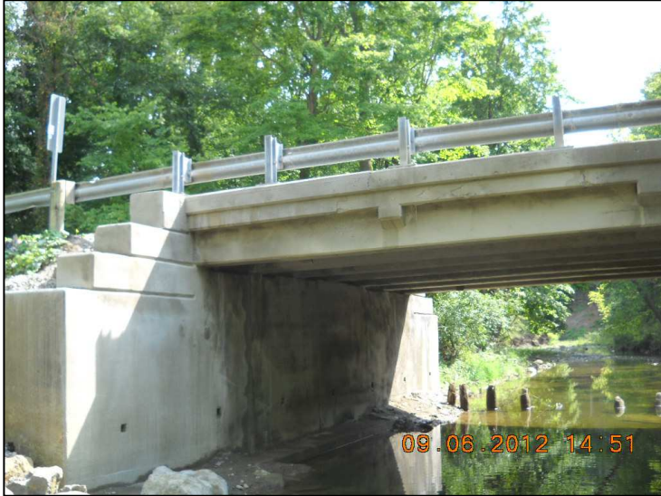
Brush Road Guniting Repair
