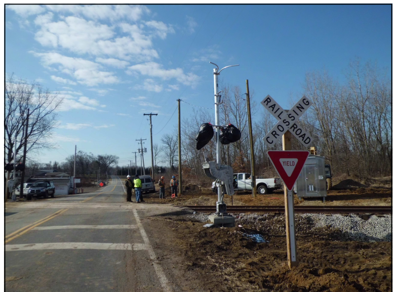
Installing lights and gates at a railroad crossing on Pressler Road
