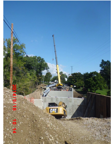
Ravenna Road Bridge Beam Setting
