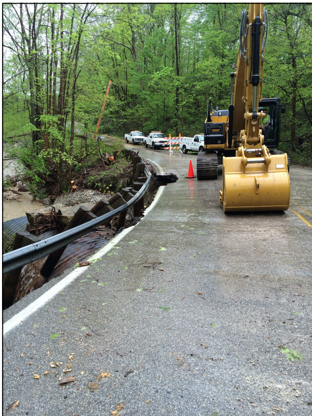
Revere Road and culvert damage
