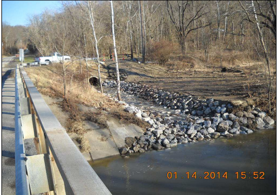
Highland Road Bridge Drainage Improvement-Replace Concrete Gutter with Limestone Rip-Rap
