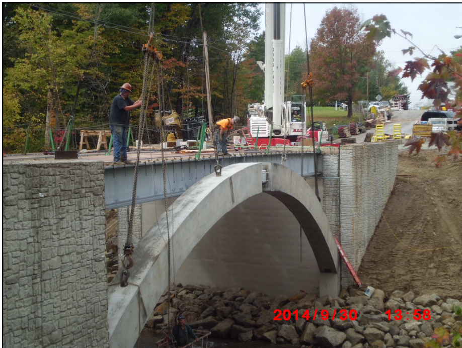
Setting the arches Ravenna Road Bridge Over Tinker's Creek
