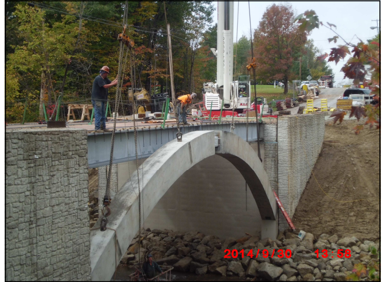
Ravenna Road Bridge over Tinker's Creek Arch Setting
