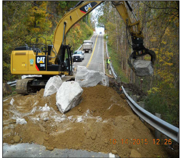
Revere Road landslide repair
