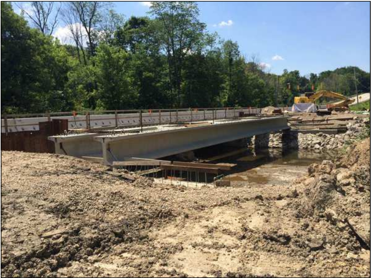
Ravenna Road Bridge over Tinker's Creek beam setting
