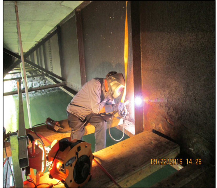
Front Street Bridge Steel Cross Frame Repair
