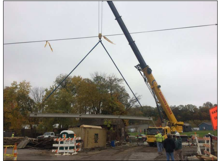
Bank Street Bridge Beam Setting
