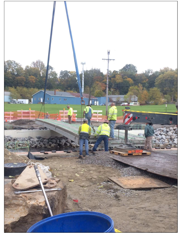
Bank Street Bridge Beam Setting
