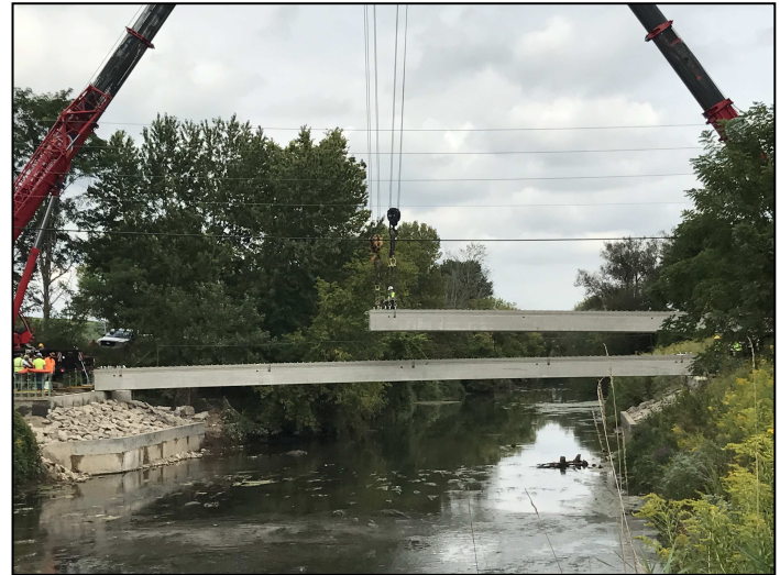
Vanderhoof Road Bridge Beam Setting
