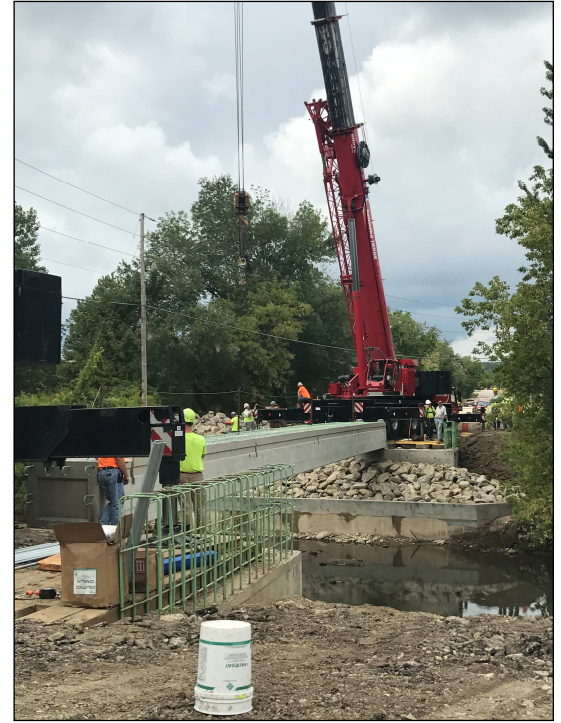
Vanderhoof Road Bridge Beam Setting
