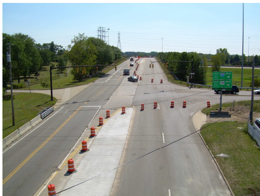
South Main Street, Phase IV—Construction is now complete.
