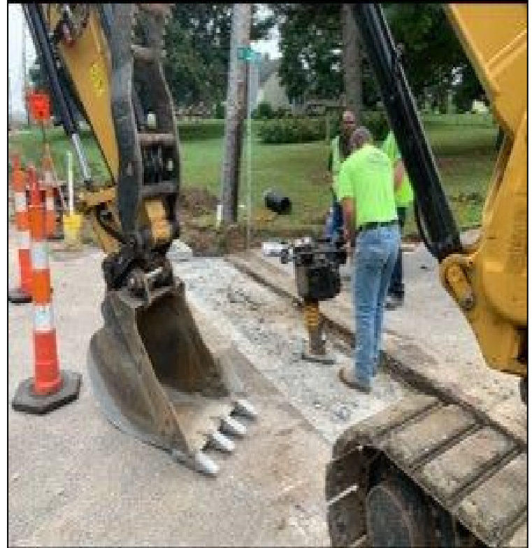
Killian at Conlin Culvert Replacement
