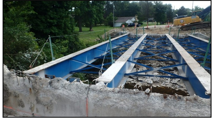
Highland Road Bridge Rehabilitation Project
