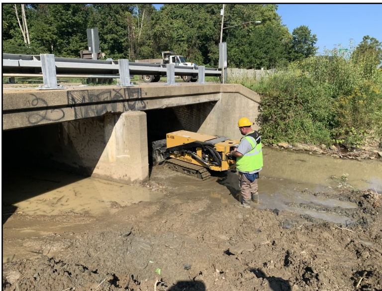
Riverview Road Bridge over Columbia Run
