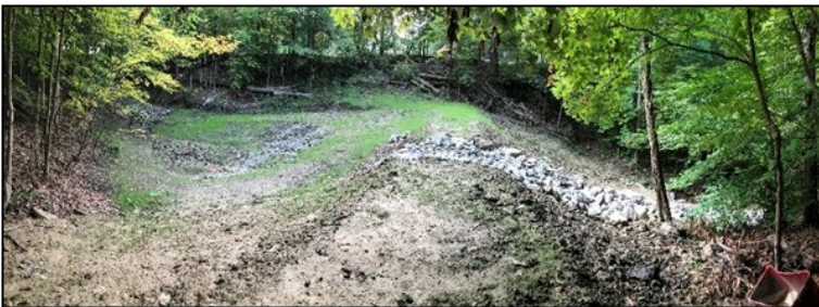
Bath Country Estates Dam Repair
