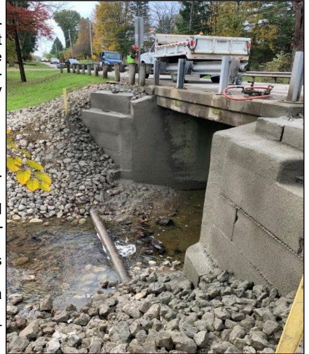
Jacoby Road Bridge Repair
