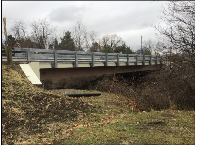
Completed Highland Road Bridge Rehabilitation Project
