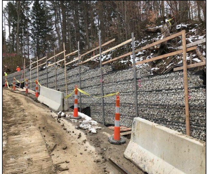
West Bath Road Landslide Repair—Retaining Wall
