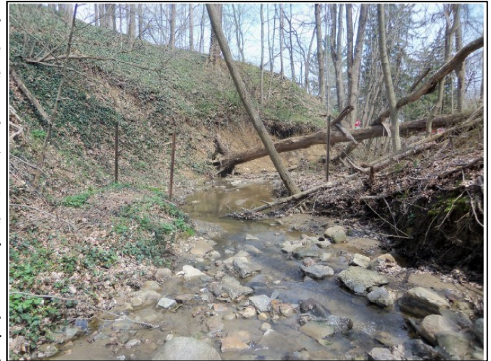
Erosion near Wye Road
