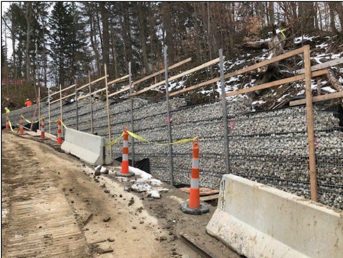
West Bath Road Landslide Repair
