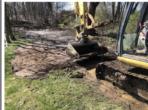
Photograph 5 (April 8, 2020). The access route was restored as the equipment was removed offsite.
