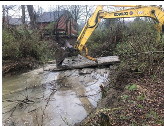
Photograph 2 (April 7, 2020). Timber mats were used to provide access into the stream.
