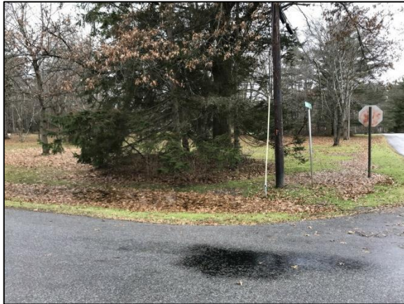
Figure 15: Culvert across Partridge Lane with landscaping rocks and driveway on left
