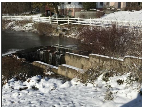
Figure 74: Outlet structure without protective measures
