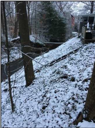
Figure 49: Steep slope and close proximity to structures
