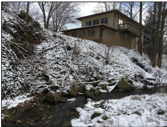
Figure 78: 4023 Shaw Road, where house may only be ~10 feet from the top of a potentially failing bank
