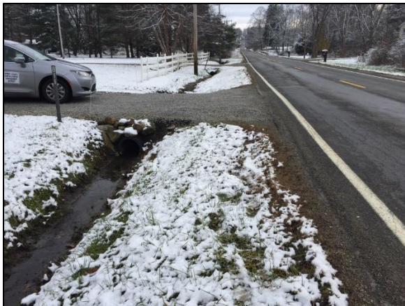
Figure 32: Driveway and existing swales on Medina Line Road (looking south)
