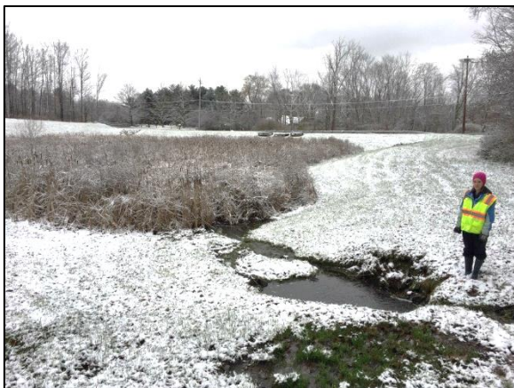
Figure 25: Tippy Run inlet and cattails covering bottom of Solar Cir basin
