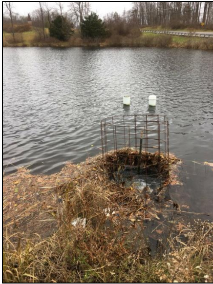
Figure 24: Outlet control structure at Ghent Road basin
