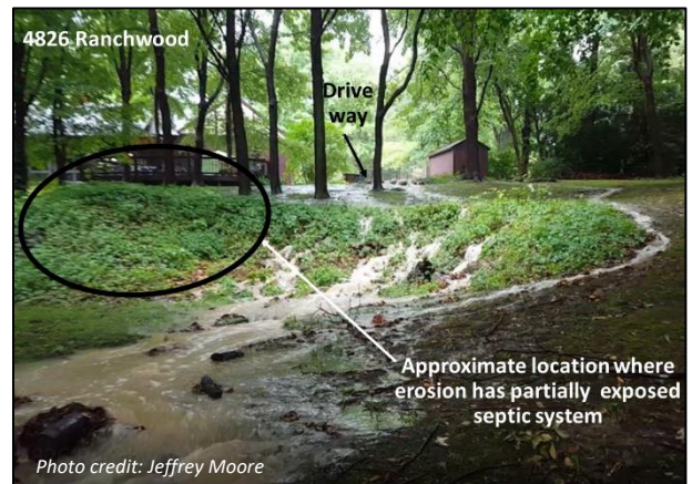
Figure 34: Flooding looking from backyard with partially exposed septic location identified
