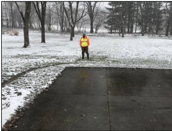
Figure 62: Resident complaint of wet spots that are slow to drain in yard.
