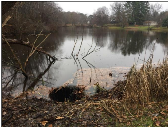
Figure 23: Outlet control structure at Goodrich Lake Dam
