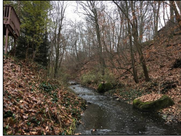
Figure 77: 2364 Berrywood Drive with encroaching deck and house on top of opposite bank
