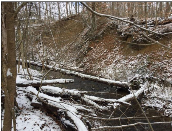
Figure 50: ~40-ft tall near vertical bank with mass wasting and tree loss
