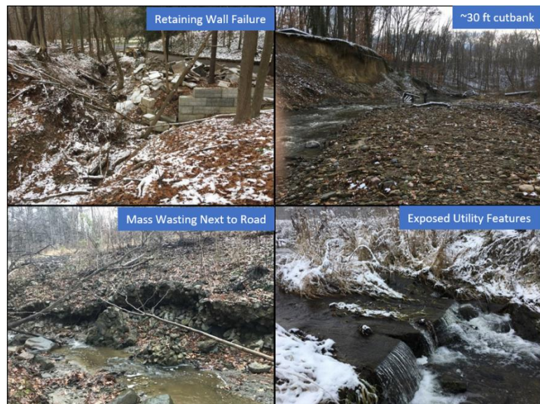
Figure 2: Hydromodification and its effects along Yellow Creek and its tributaries
