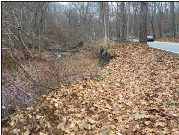
Figure 56: Revere Run valley in close proximity to Revere Road
