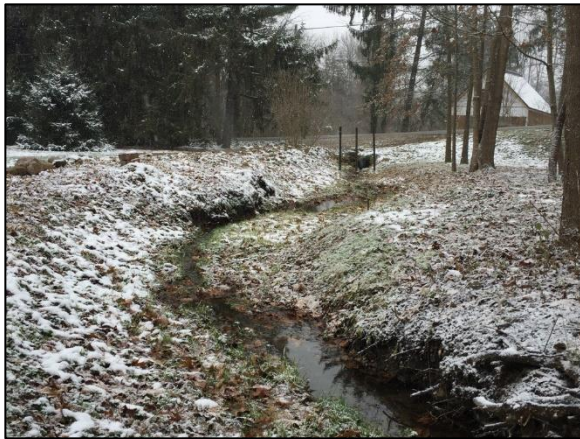
Figure 14: Culvert across Partridge Lane with landscaping rocks and driveway on left
