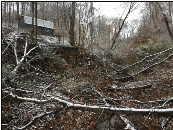
Figure 53: Extensive tree loss along Merrill’s Run with shed at top of bank
