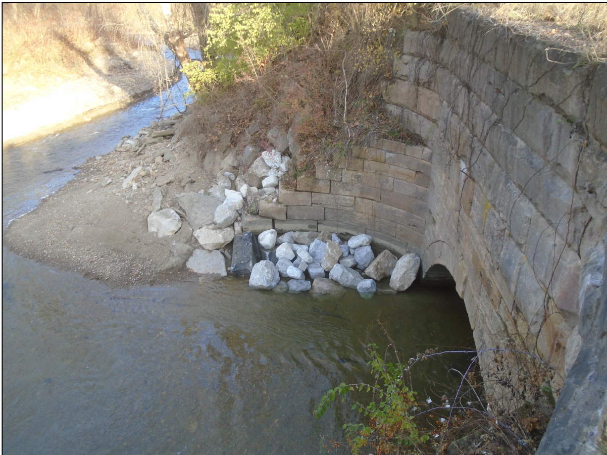
2018 Riverview Road Bridge Scour Mitigation—SCE's oldest bridge
