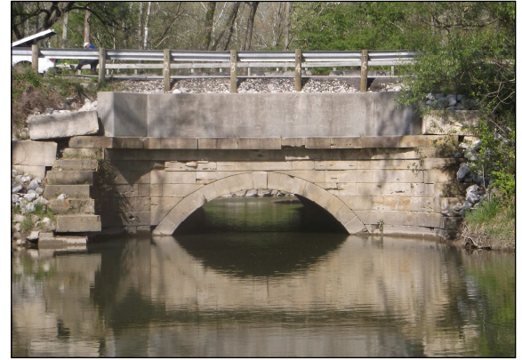
Riverview Road Stone Arch Bridge
