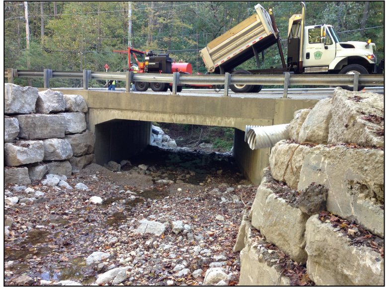
Martin Road Bridge—Erosion Control Project
