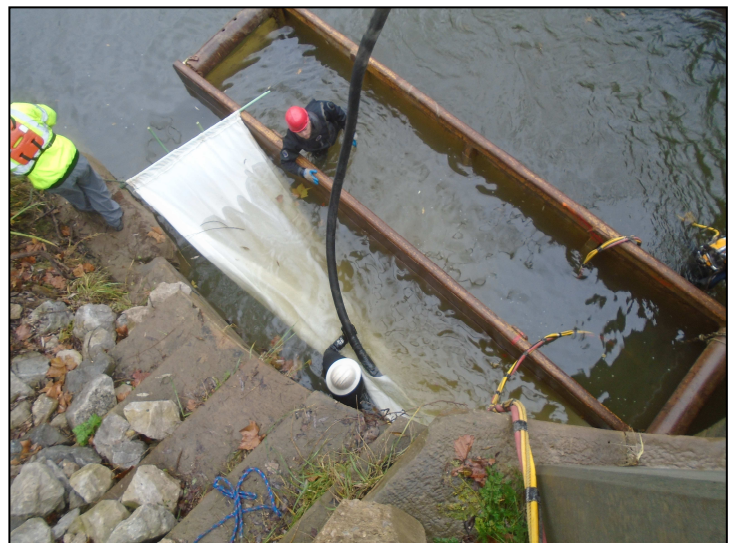
Riverview Road Bridge over Yellow Creek Scour Mitigation
