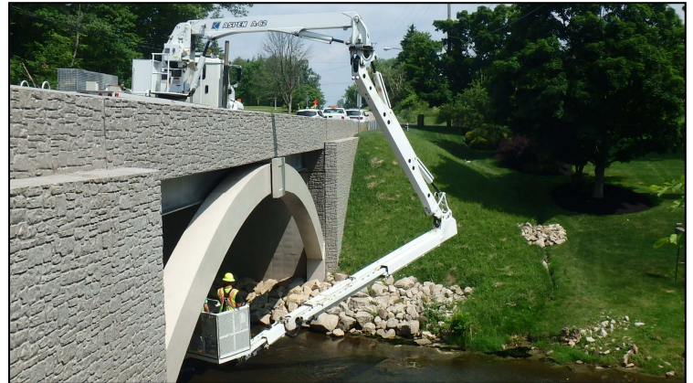
Ravenna Road Bridge over Tinker's Creek—Snooper Truck Inspection
